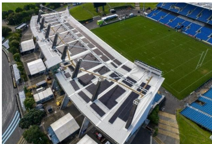
Figure 5: New solar panels installed at Go Media Stadium
