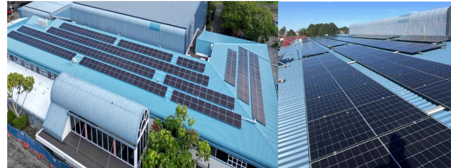
Figure 4: Allan Brewster Leisure Centre now uses solar photovoltaic cells to help meet its energy needs
