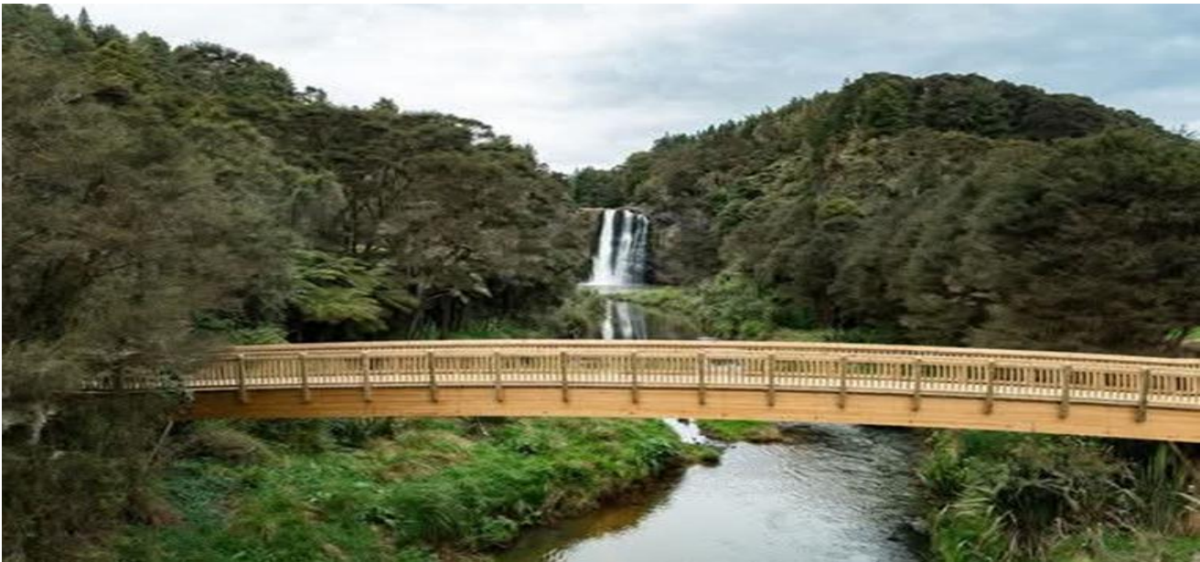
Hūnua Falls bridge replaced in August 2024
