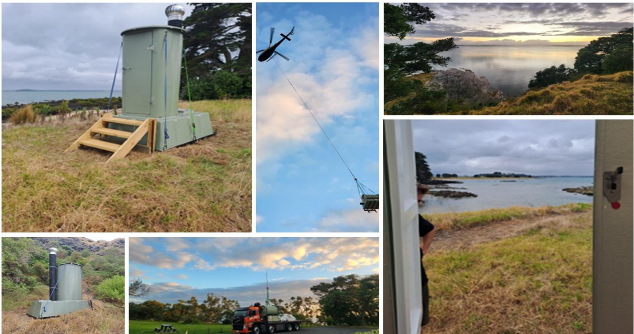
Installation of new toilets on Motukorea / Browns Island
