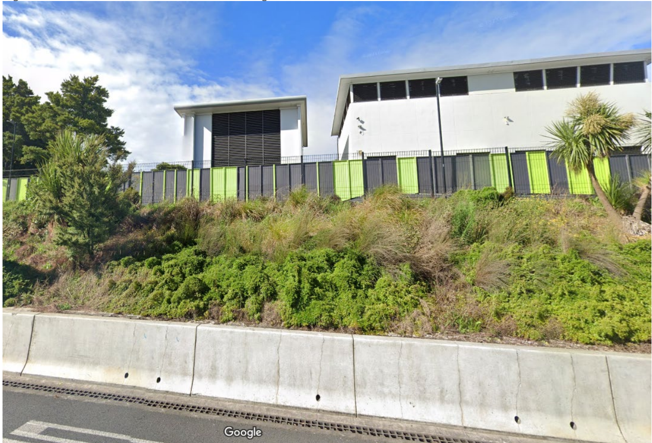
Figure 8: Timber nose wall at Te Atatū interchange on SH16
