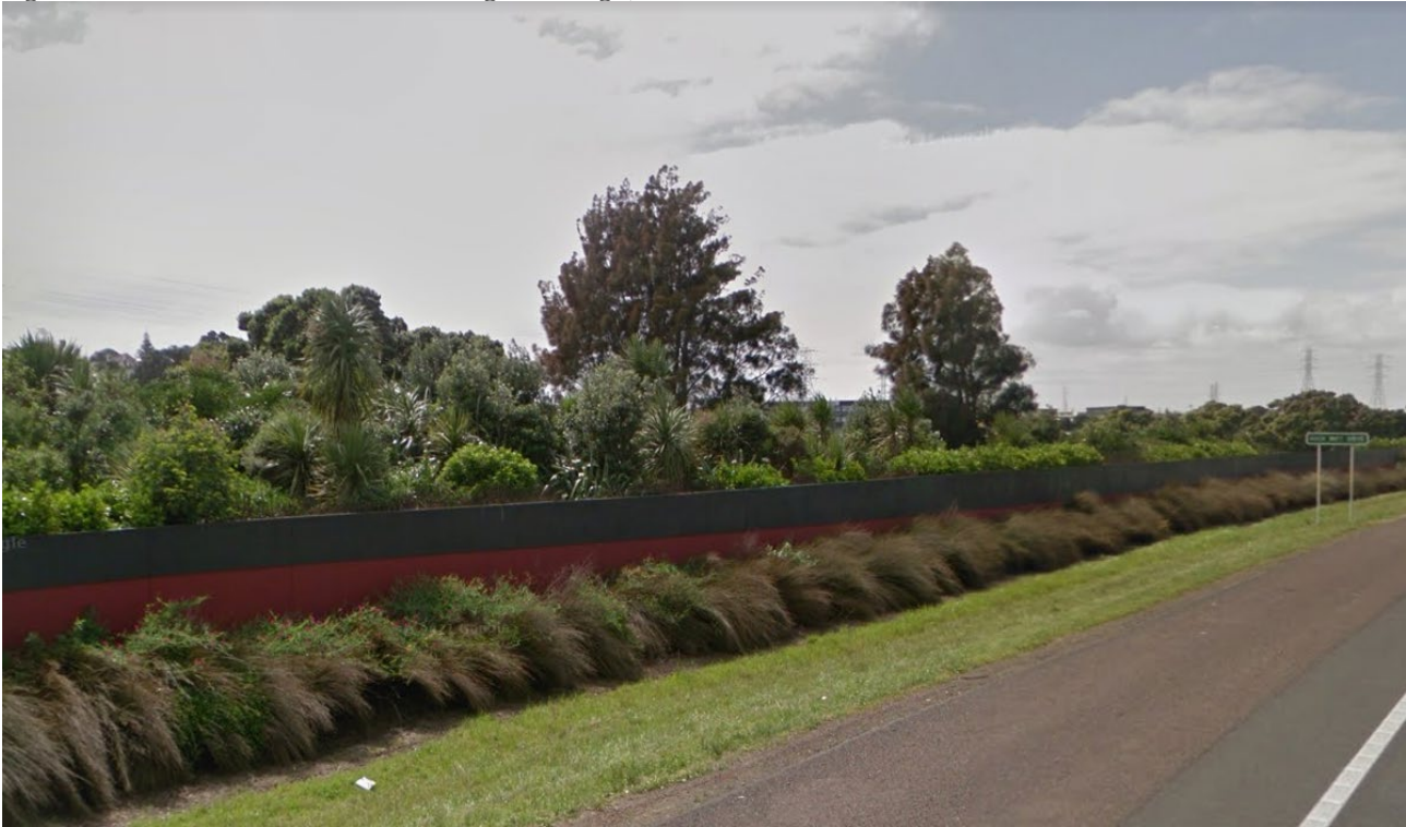
Figure 7: Timber noise wall along Northern Busway on SH1, constructed prior to 2009
