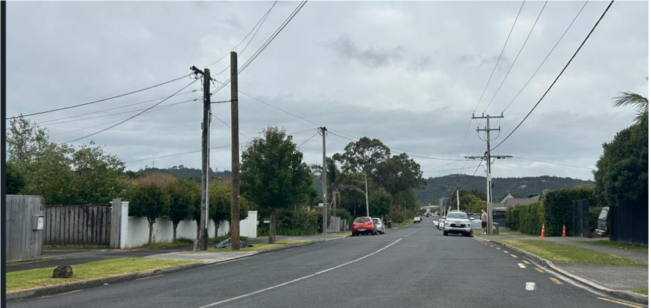
Figure 2.10 Existing school access on Trigg Road, looking north
