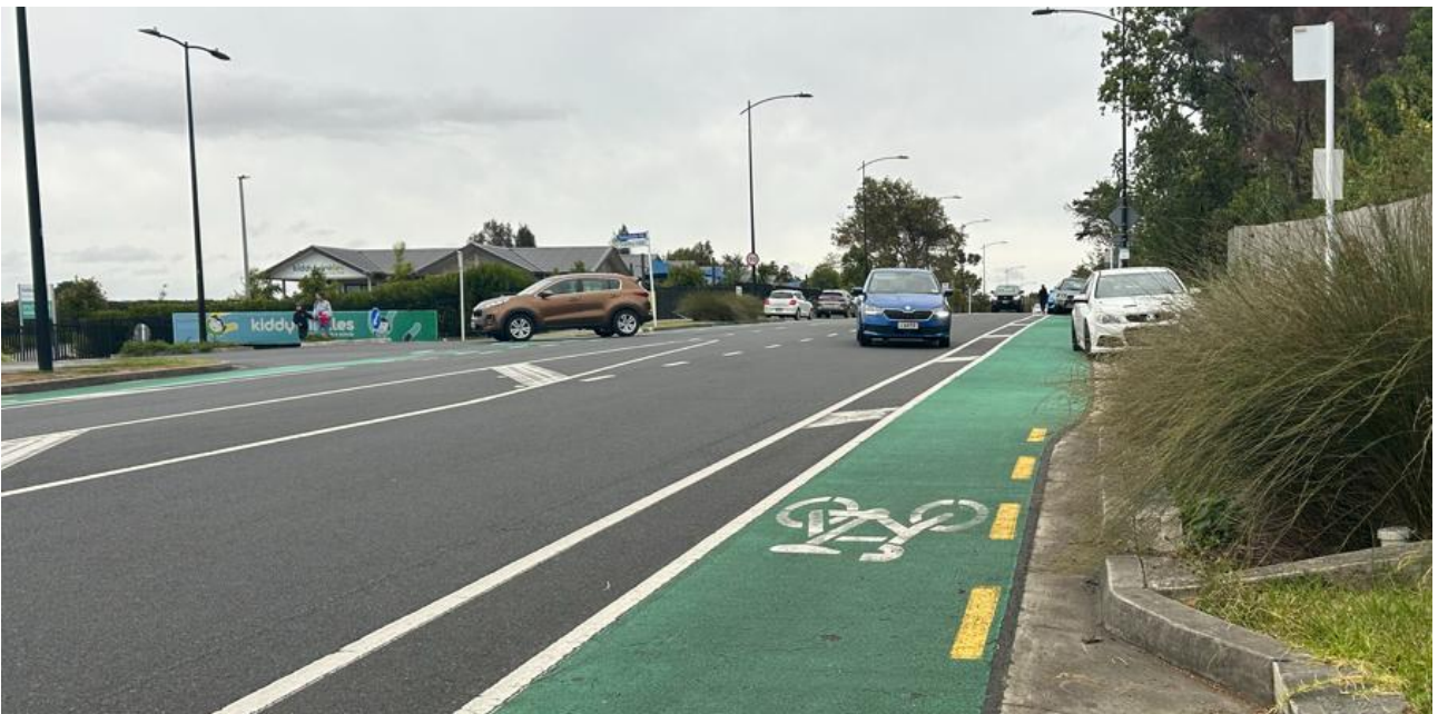
Figure 2.9 Existing school access on Station Road, looking south
