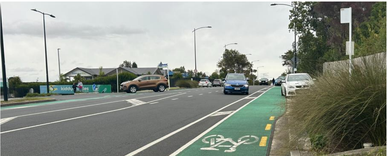
Figure 2.16 Potential location for a PUDO Exit at the northern end of the site frontage on Station Road, looking south
