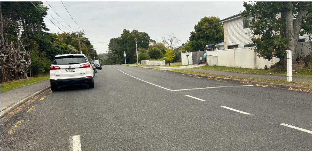
Figure 2.11 Existing school access on Trigg Road, looking south
