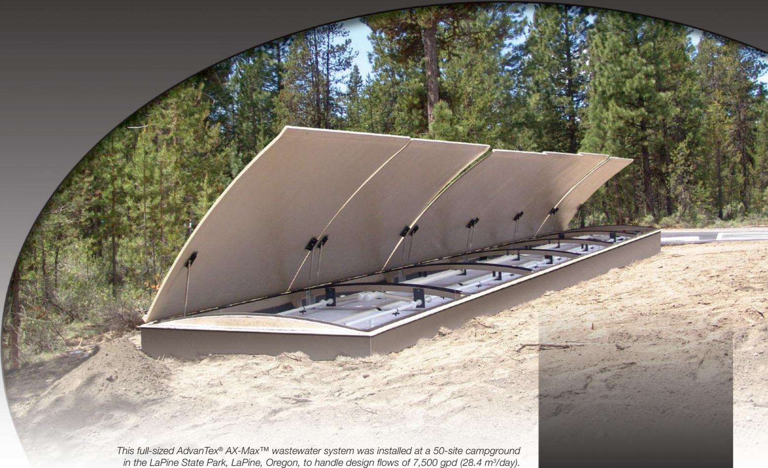
*This full-sized AdvanTex® AX-Max™ wastewater system was installed at a 50-site campground in the LaPine State Park, LaPine, Oregon, to handle design flows of 7,500 gpd (28.4 m<sup>3</sup>/day).*
