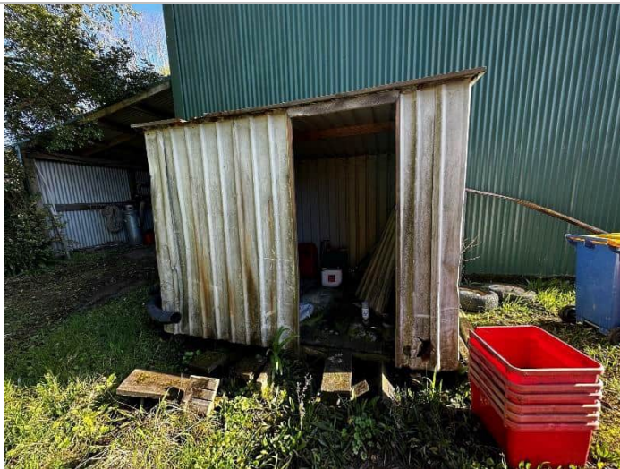
Photo 5: Small metal shed located to the southwest of the large shed (pictured in the background). Small volumes of fuel and oil observed in the small shed.
