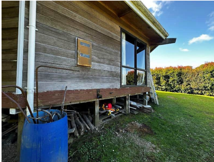
Photo 9: Construction materials (timber, PVC pipe and piping) observed beneath the dwelling.
