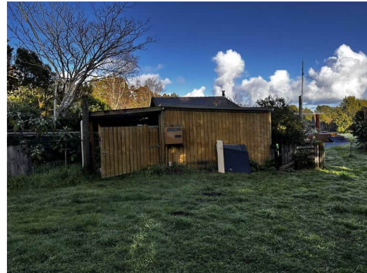
Photo 4: Shed / garage to the east of the dwelling.
