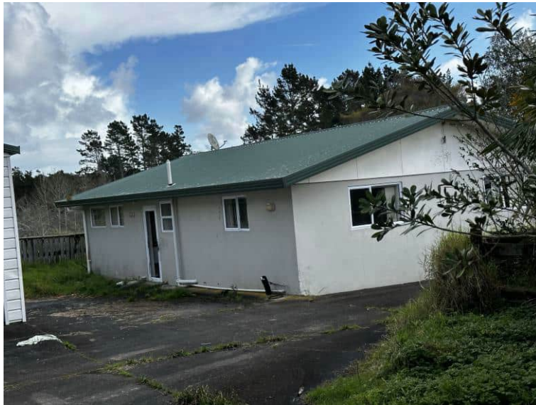
Photo 3: Granny flat in the south-eastern corner.
