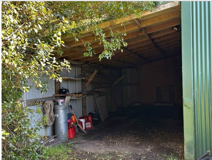
Photo 7: View of entrance to the lean-to shed. Small volumes of oils and fuels were stored next to the entrance of the lean-to, on the earthen floor.
