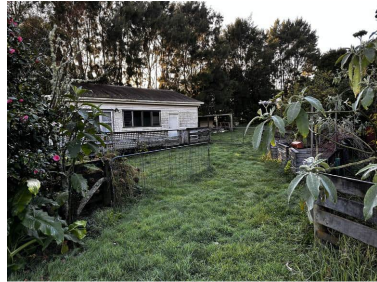
Photo 2: Building positioned on northern site boundary, in the eastern corner of the site.
