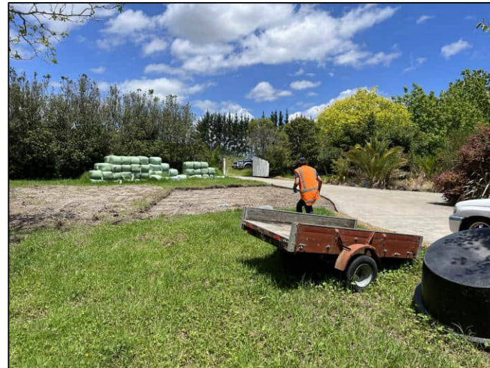
Photo 4: Former building footprint in southeast portion of site, and location of fill material.
