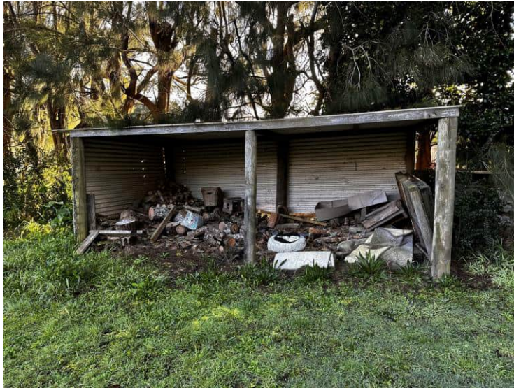
Photo 5: Wood storage shed.
