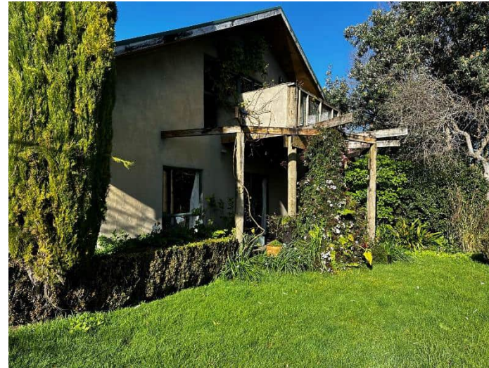
Photo 10: Potential living quarters at the northern end of the large shed.
