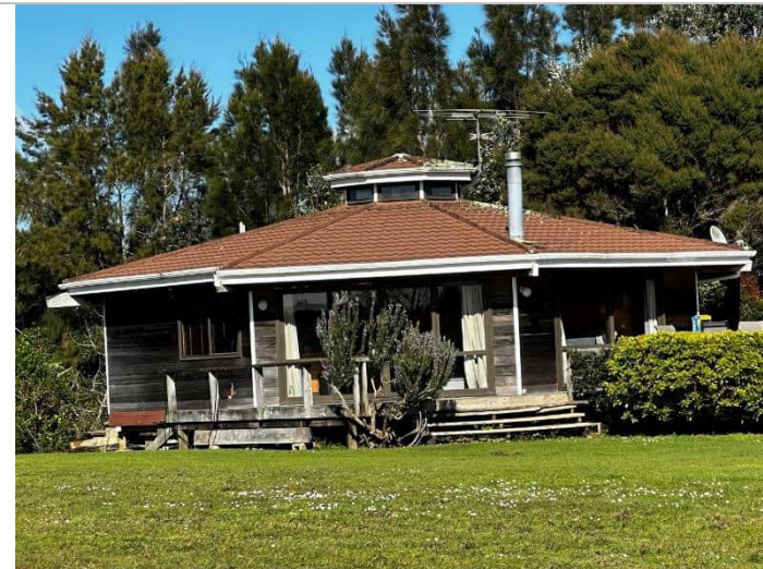
Photo 8: View of southernmost timber clad dwelling, located in the western portion of the site.
