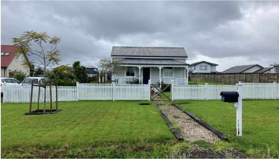
Figure 7: Clarks Lane workers cottages.
