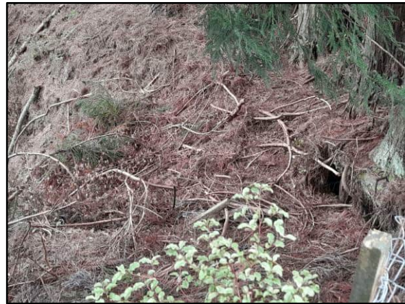
Photo 4: Shallow failure scarp on north-western slope
