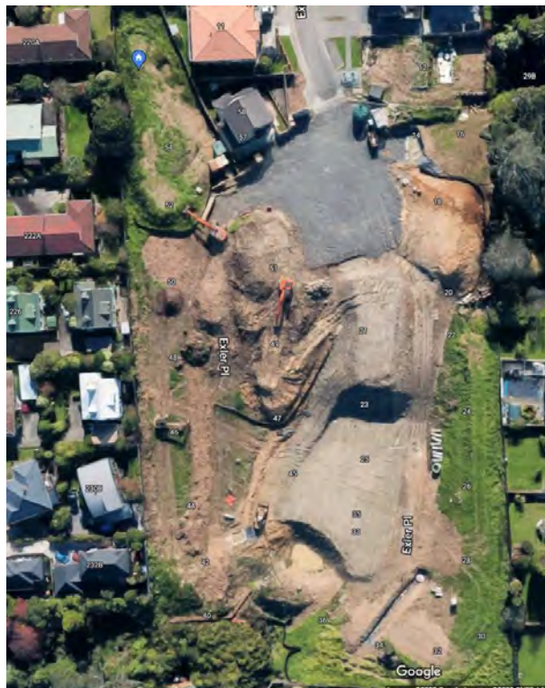
An aerial image showing the extensive earthworks and infrastructure build during the land conversion from farm land into the current development (Source: Google)
