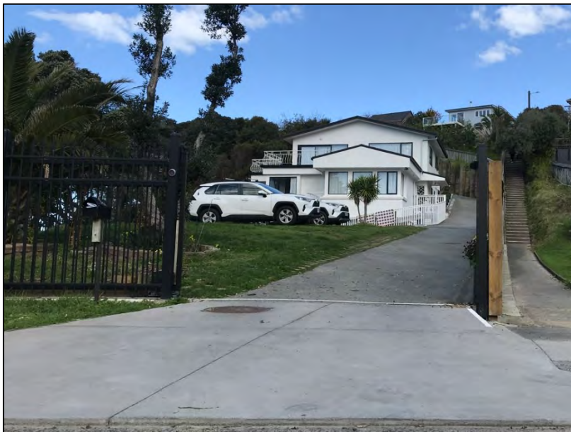
Figure 6: Existing site (with upgraded accessway), as viewed from street frontage.
