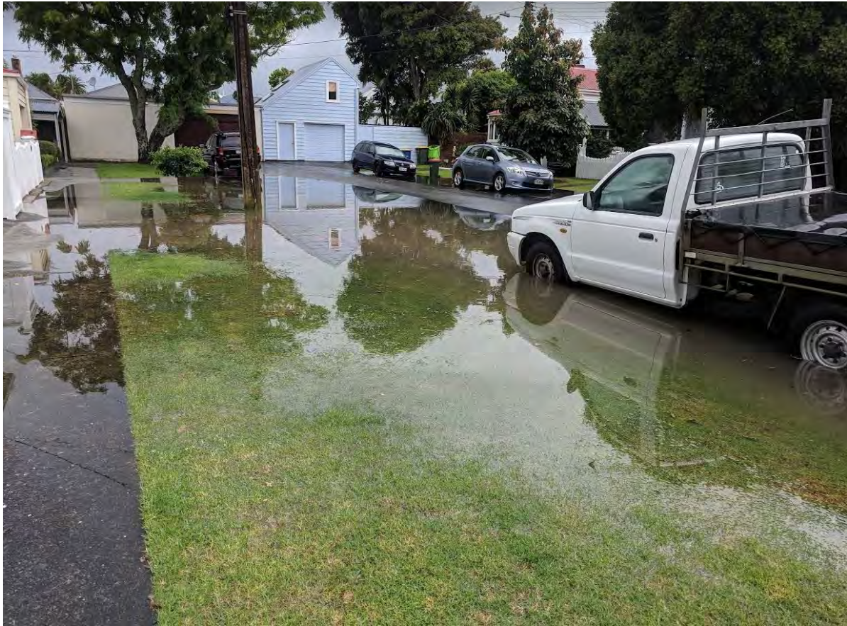
Image 3 – 25 December 2018 flooding in front of 5 & 7 Kapai road Devonport
