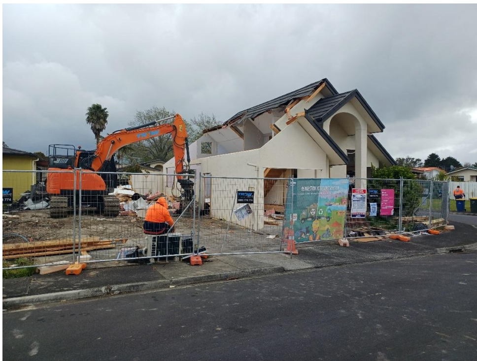
Mechanical deconstruction in action
