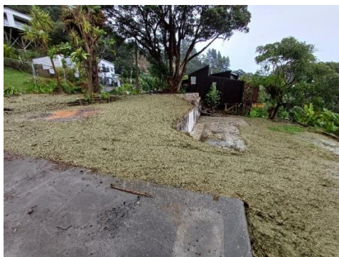
Concrete wall and slab left in place as acting as retaining (grass is still to establish)
