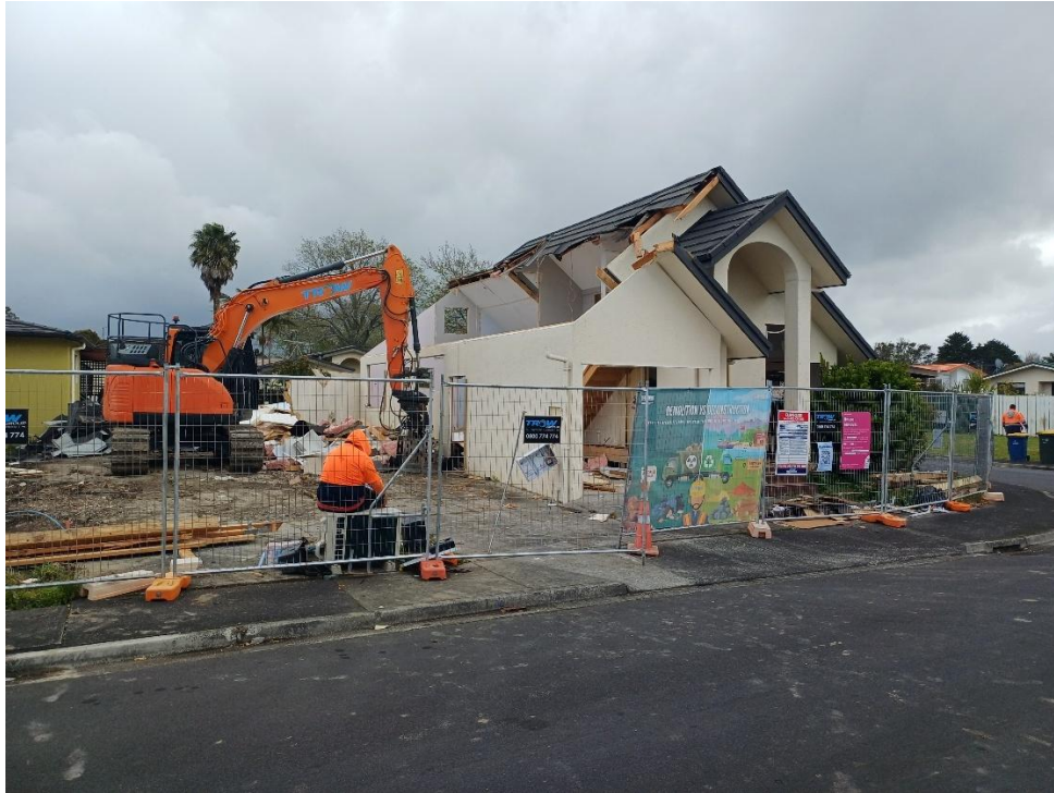
Mechanical deconstruction in action
