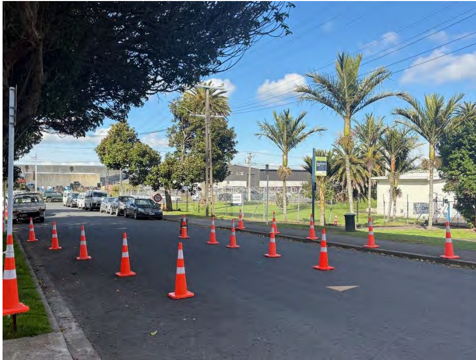
Figure 2: Streetscape view along Spring Street looking south-west towards the WTP.
