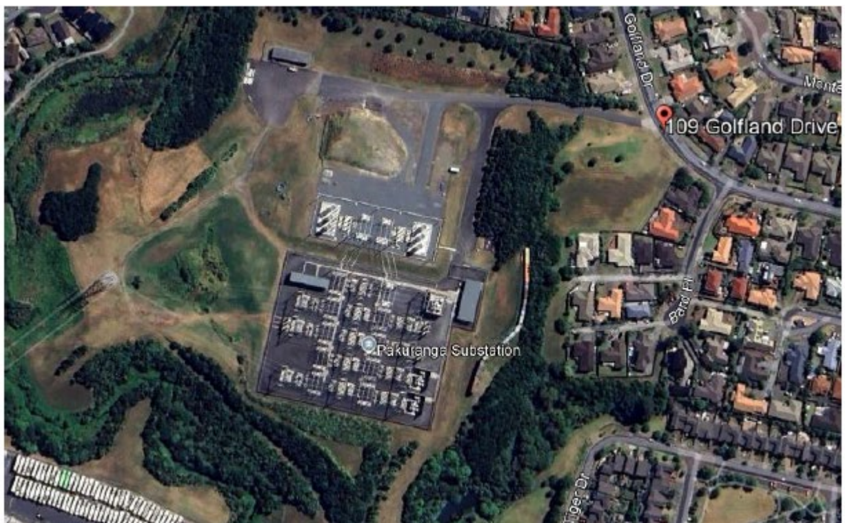
Figure 2 – Updated aerial imagery 2024 - shows the new switchyard and the noise buffer containers installed on the eastern boundary [source - AEE]
