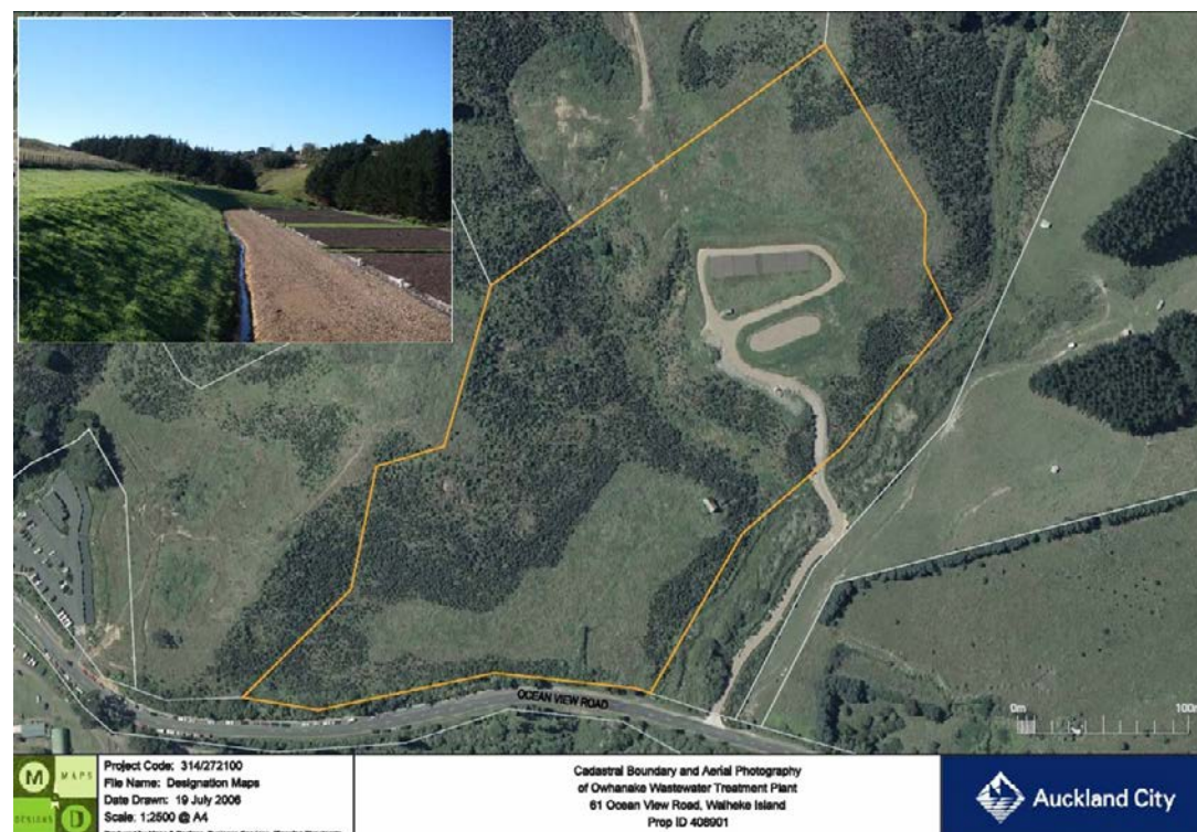
Figure 5a: Rural wastewater treatment plant requiring periodic re-consenting
