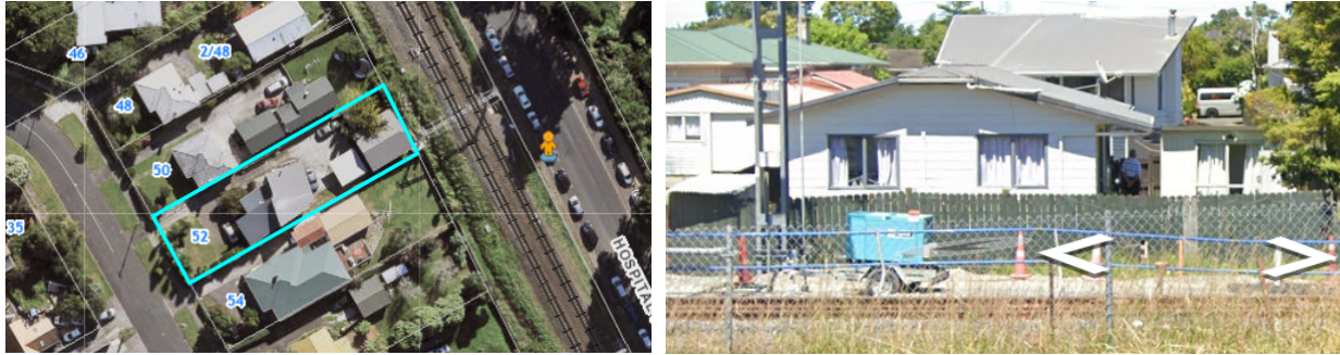
Figure 4-1: Rear of 52 Rosella Road as seen on from Hospital Road (source Google Street View 2025)
