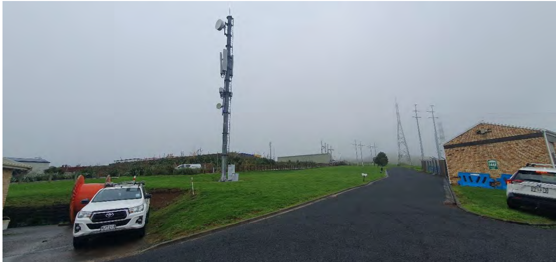
Figure 5: Counties Energy Substation viewed from Bombay Substation
