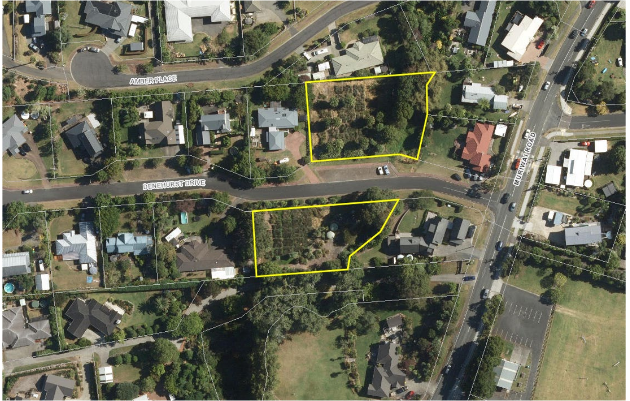
Figure 1: Location of the Denehurst Wastewater Treatment Plant (Source: Auckland Council Geomaps Satellite Imagery 15 May 2025)
