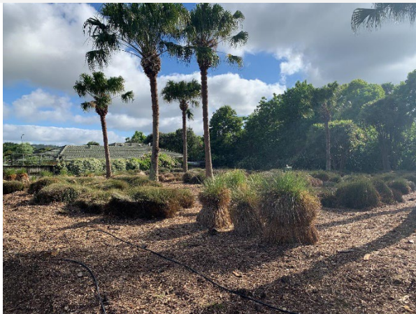
Figure 2-11: Drip irrigation field located on No.4 Denehurst Drive (Source: Aurecon)
