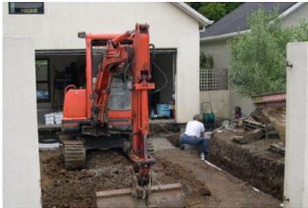
Fig.1 Excavation to design level.
