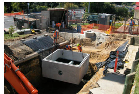
Fig.3 Sand filter chamber is lowered into the receiving pit.
