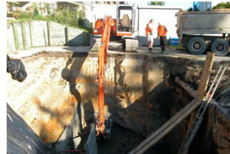
Fig.1 Excavation of chamber pit
