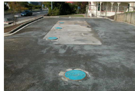
Fig.5 Completed sand filter. Blue lids show the access locations.
