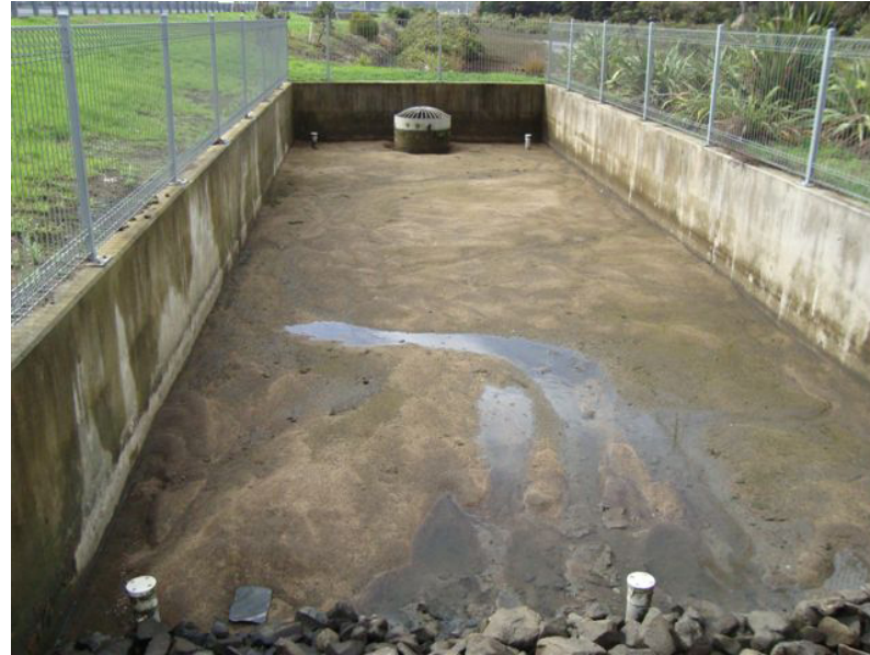
Open sand filter constructed in-situ (Photo: NZTA)
