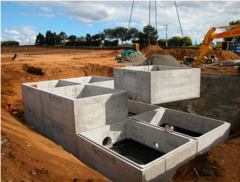
Pre-cast sand filter chambers being installed (Photo: Hynds Environmental Ltd)
