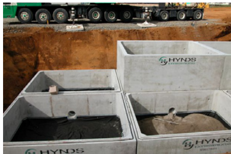
Fig.4 Showing filter media installation
