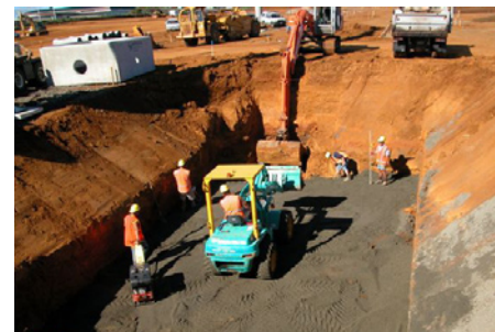
Fig.2 Basecourse installation and compaction before sand filter installed on the pit
