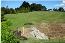
Fig.9 Dewatering control measures (also helps to control sediments) at the outlets during construction
