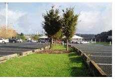
Fig.8 Constructed swale. Picture shows curb cuts as inlets, established dense grass and plants (North Harbour Stadium)
