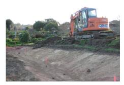
Fig.5 Excavation, preparation of side slopes to form channel
