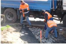
Fig.6 Construction of inlets with erosion protection
