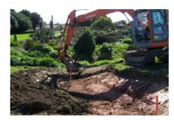
Fig.7 Preparation of top soil layer (minimum 100mm) for planting
