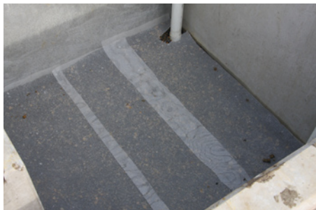
Fig.2 Root barrier installed to protect underdrain
