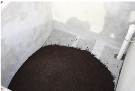
Fig.3 Backfilling of treepit, filling with soil mix
