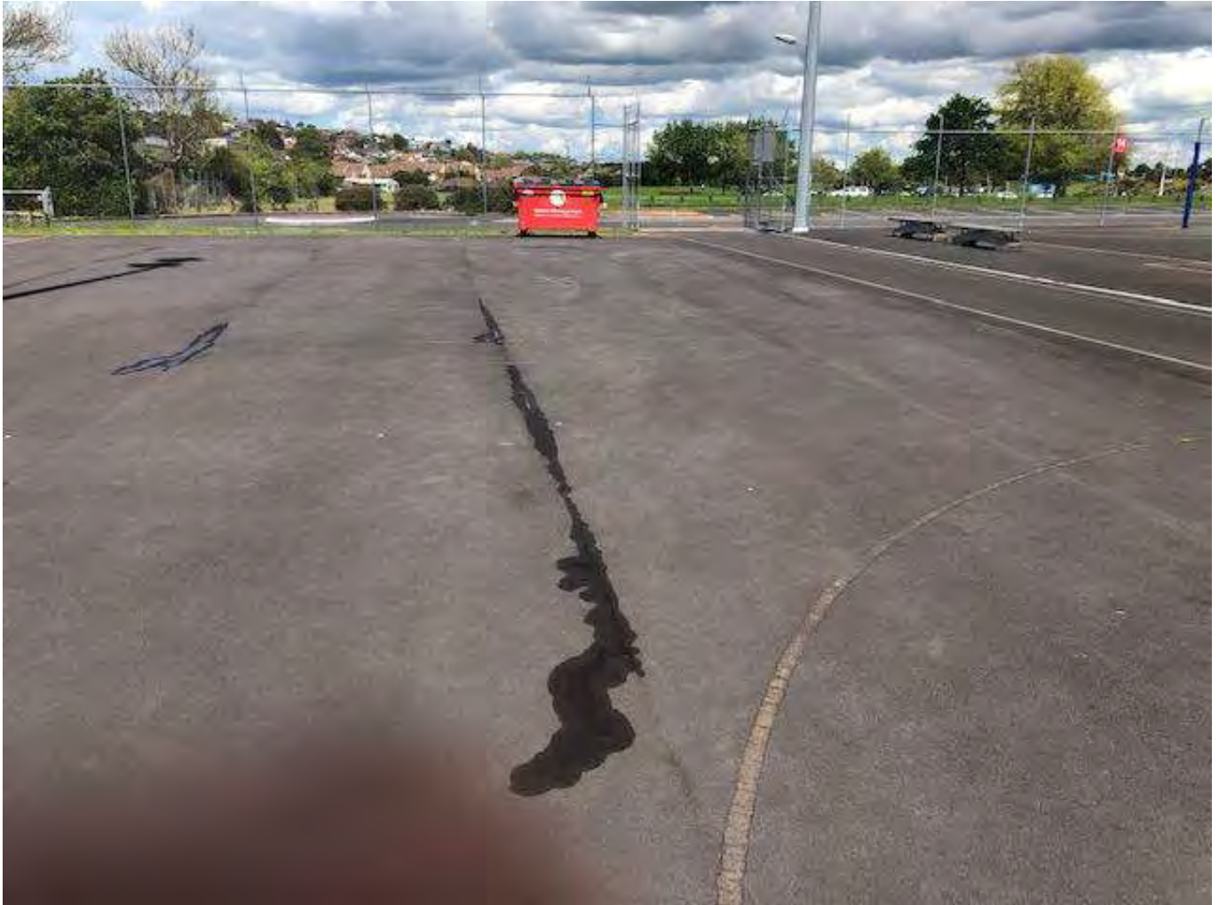
Water in the base coming out of seams
