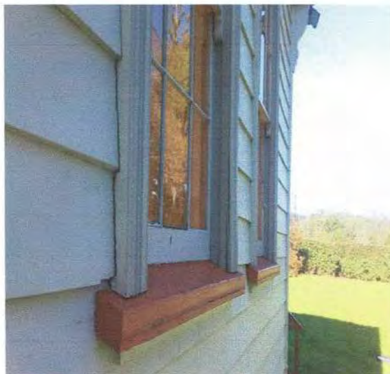
8 Window sill and scribes cracked & decayed
