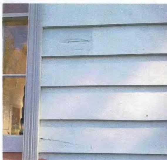
6 Exterior cladding split and decayed.
