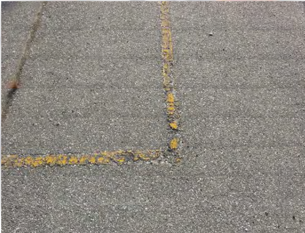
Central Otago existing asphalt condition – cracked lines, seams and very boney surface
