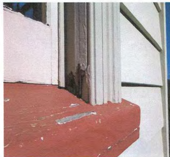
12 Timber facing and scribes to windows decayed
