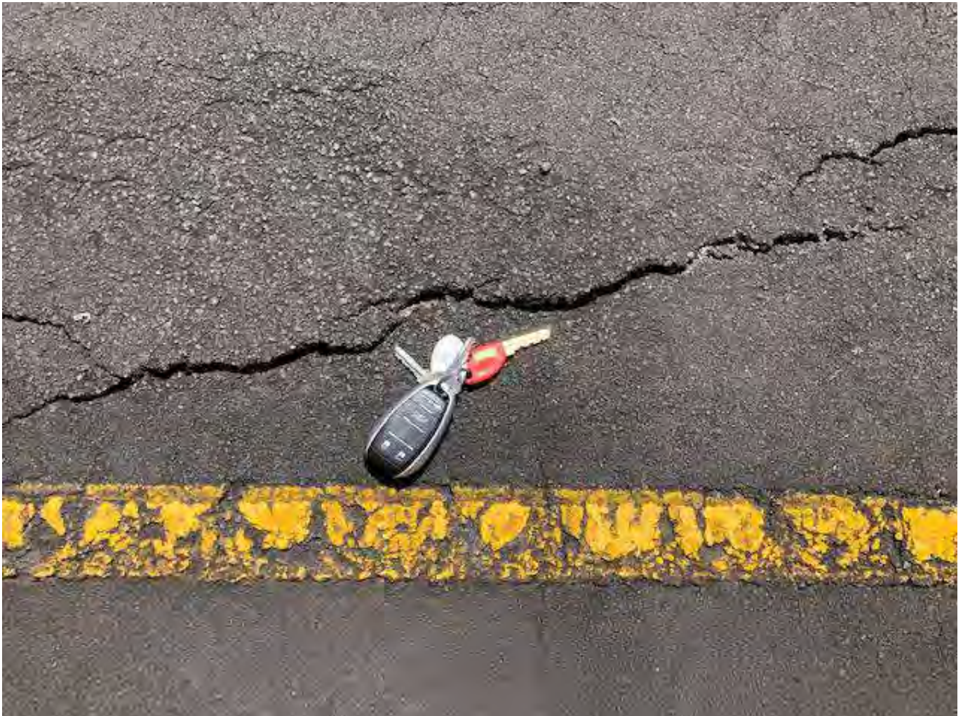
Extensive cracking within the court
