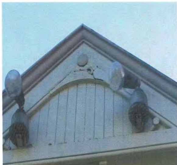
13 Gable end timber trimmer decayed.
