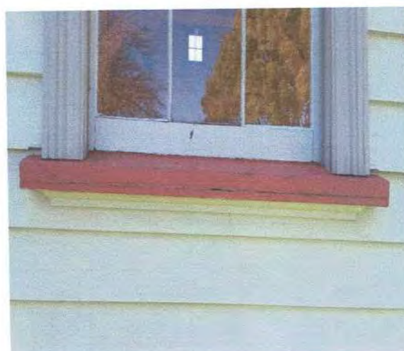
23 Window sill cracked
