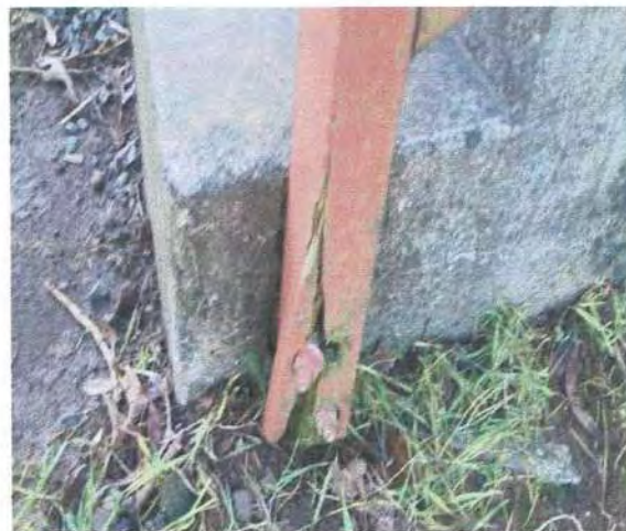
16 Handrail post decayed and bolts loose
