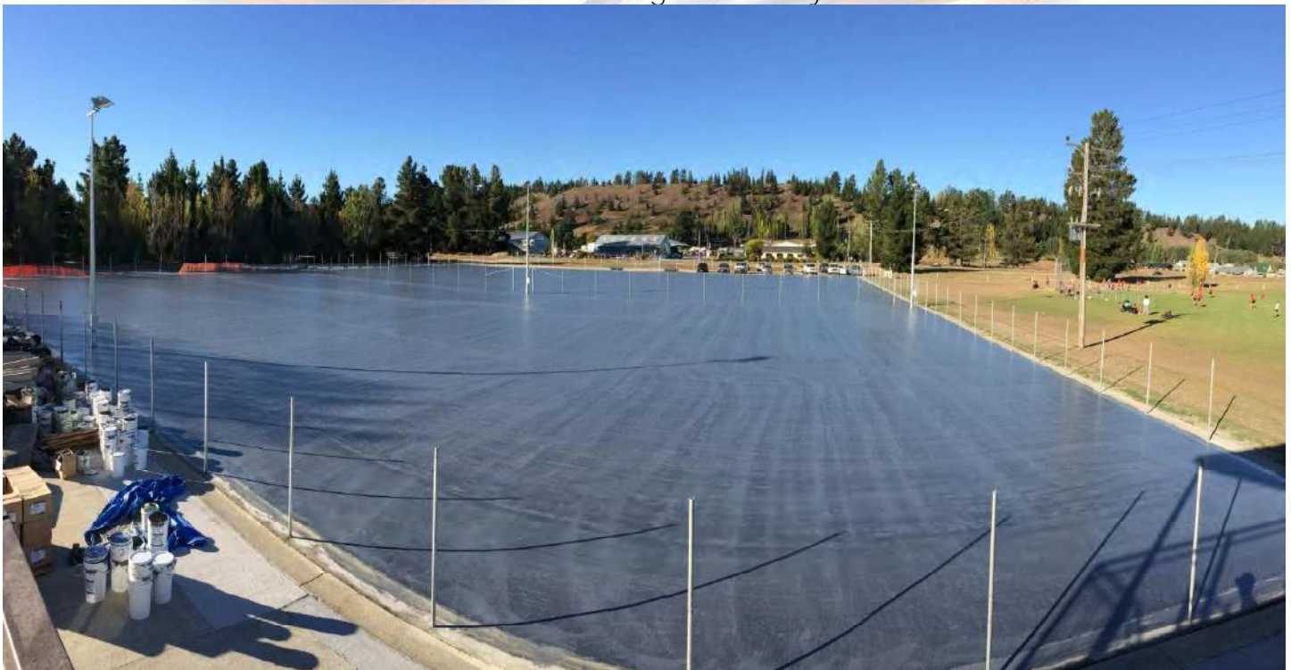
Rubber mat after two sealer coats plus tapering around mat edges
