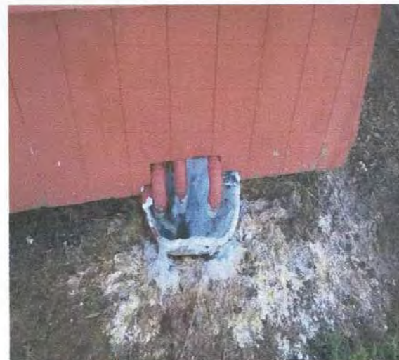
18 Gully dish blocked and grate cover missing
