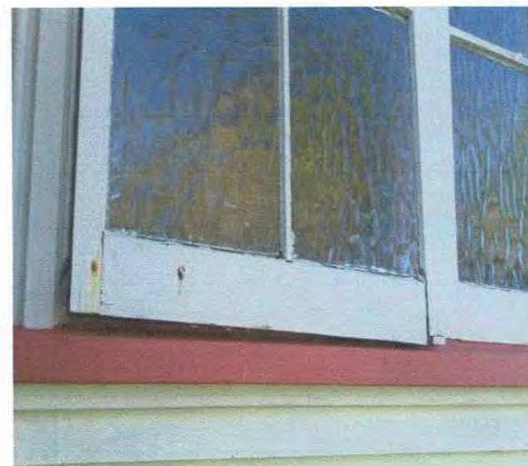
17 Window pane putty cracked and missing
