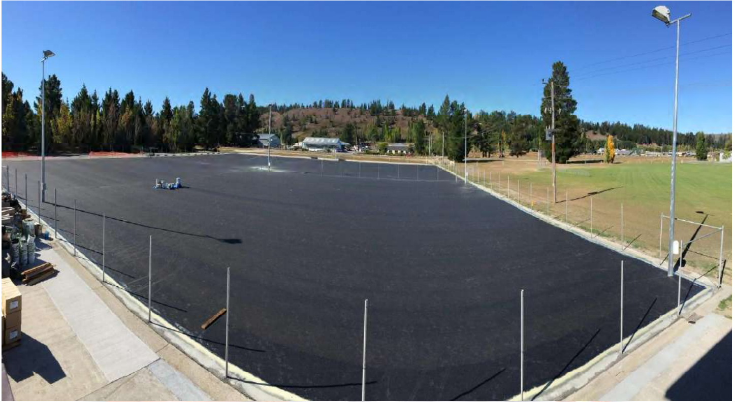
After 4mm rubber mat is glued directly to resurfaced area
