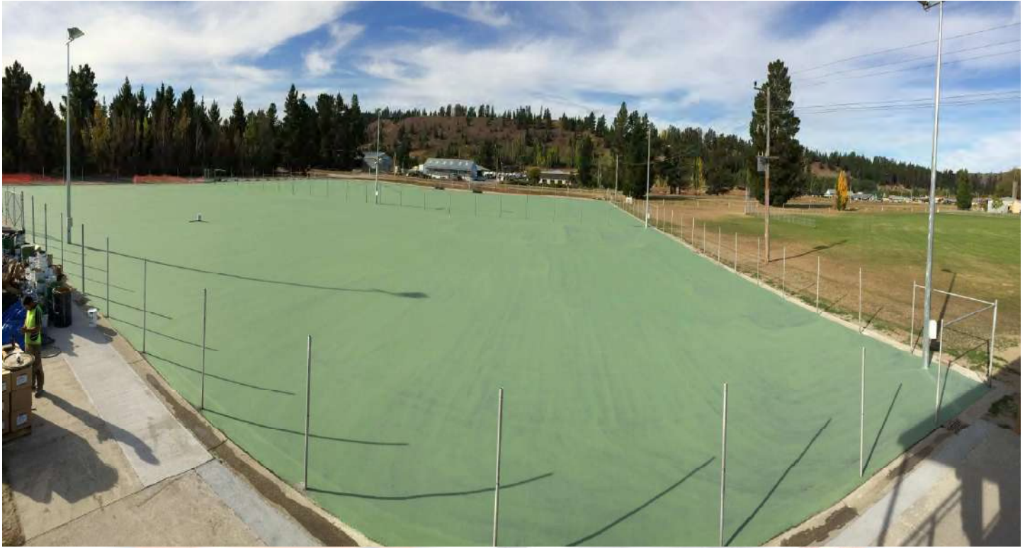
After first filler acrylic coat applied (two coats in total)
