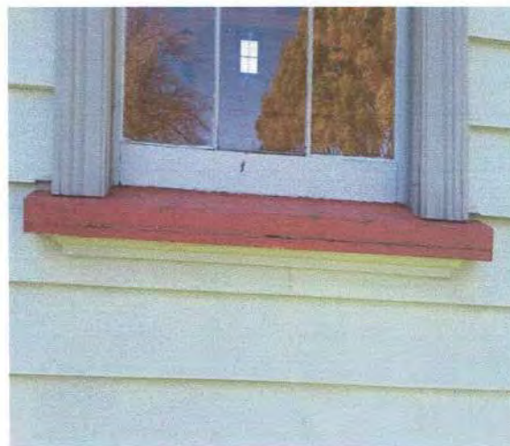
10 Window sill cracked
