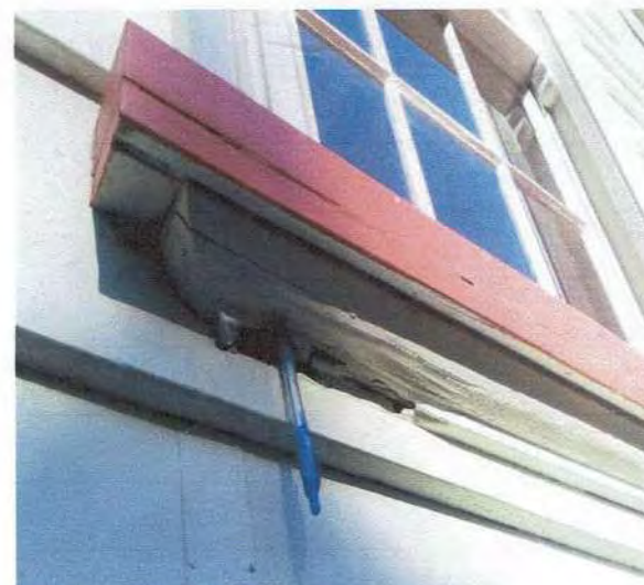
11 Timber beading under window sill decayed
