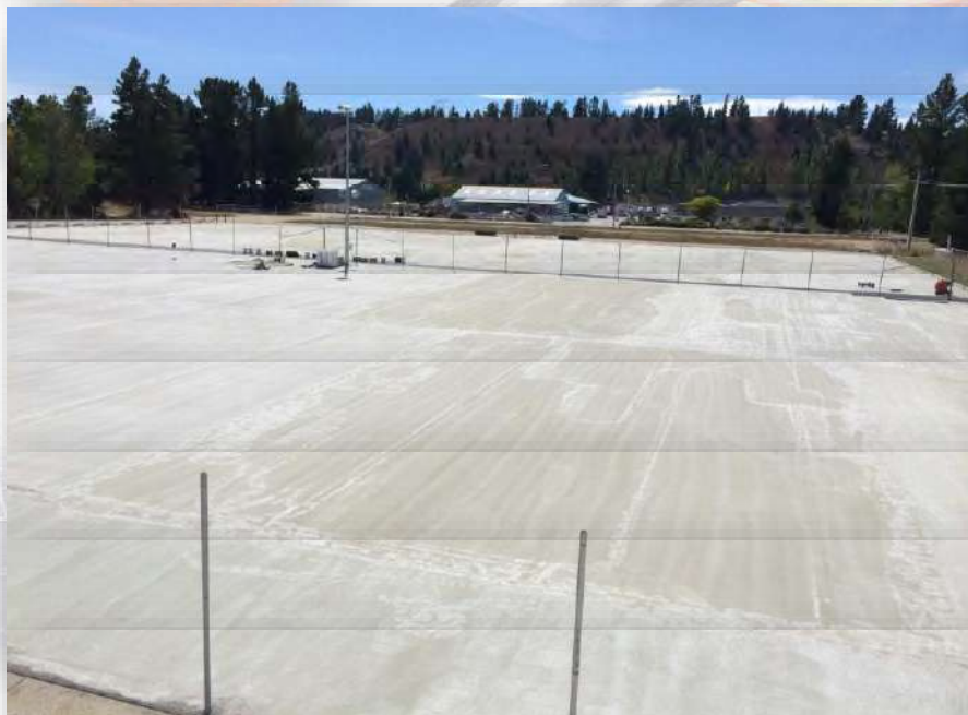
Grinding and patching of the surface, seams and lines
