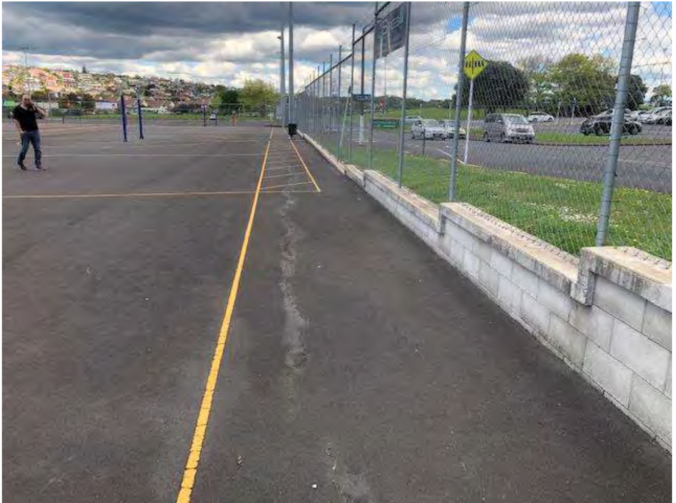
Cracked section
