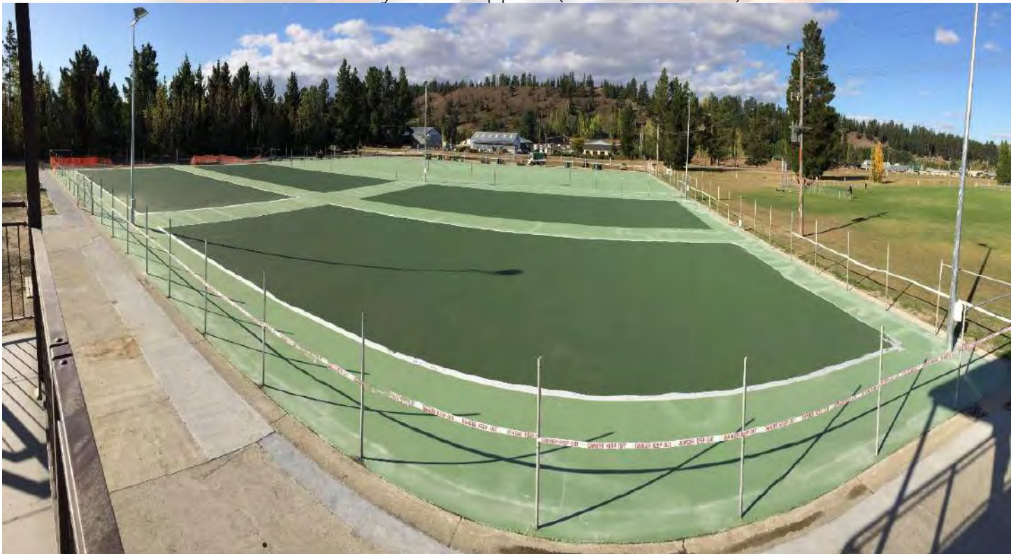
Putting the topcoat broomed surface down to internal netball courts
