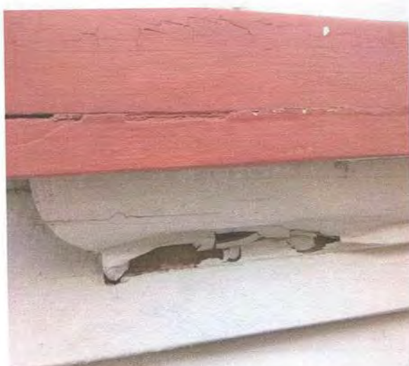
24 Window sill cracked and timber bead decayed
