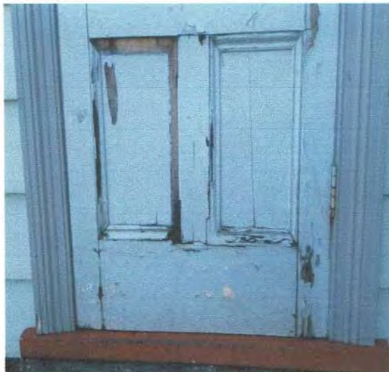
14 External on west side door decayed
