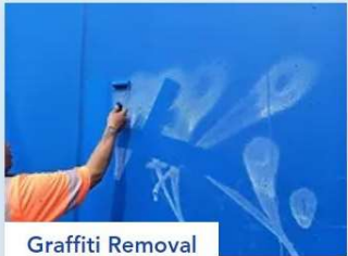
Graffiti Removal & Prevention
