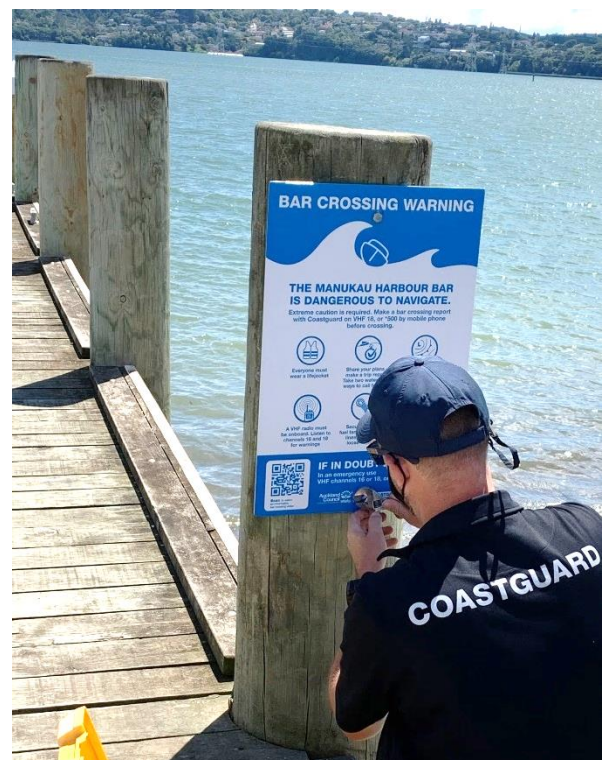
Erecting Safety Signage, Manukau Harbour
