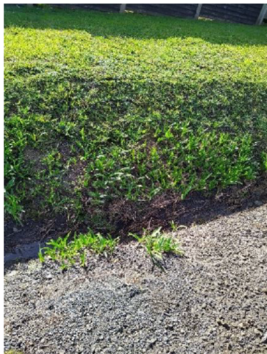
(Roadside, embankment and culvert along 67 McEntee Road)
