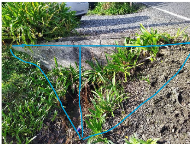
(View onto culvert and current drive way & street at 69 McEntee)
