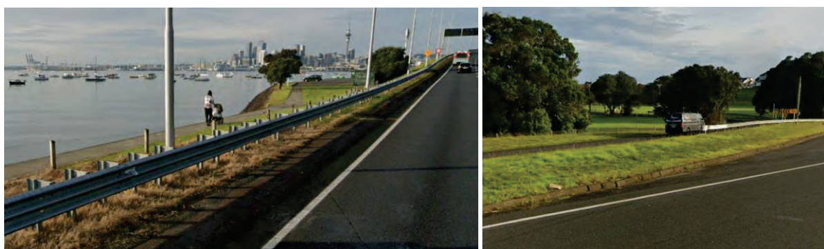
Figure 10 Low fence and direct access onto SH1 at Sulphur Beach
