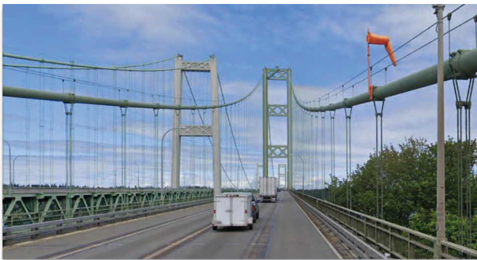
Figure 28 Windsock deployment to provide regular users with direction and strength information (Tacoma Narrows Bridge, Washington State, USA)
