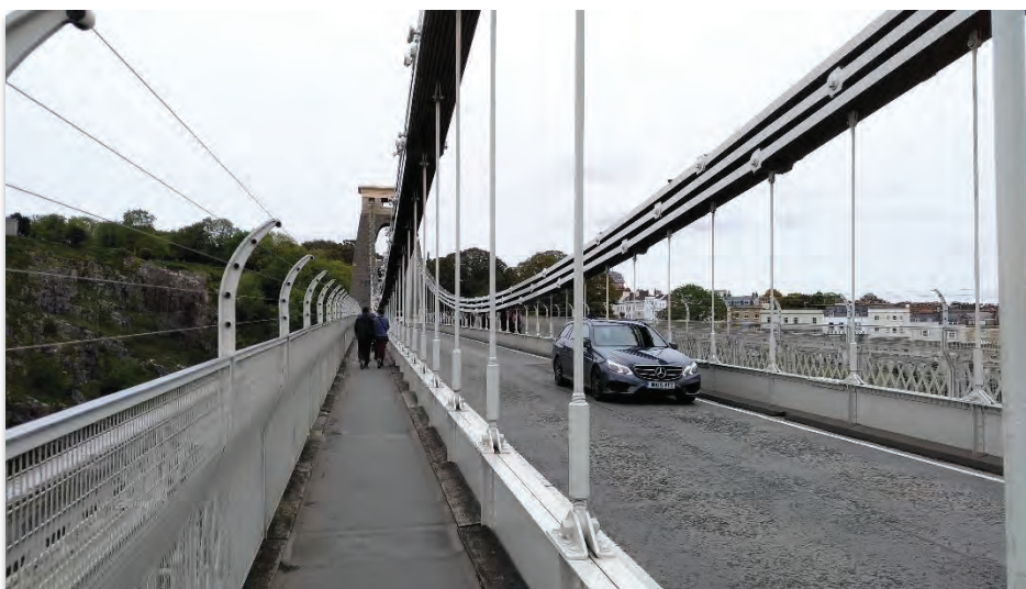
Figure 9 1998 anti-climb barriers on Clifton Suspension Bridge (1.9m height)
