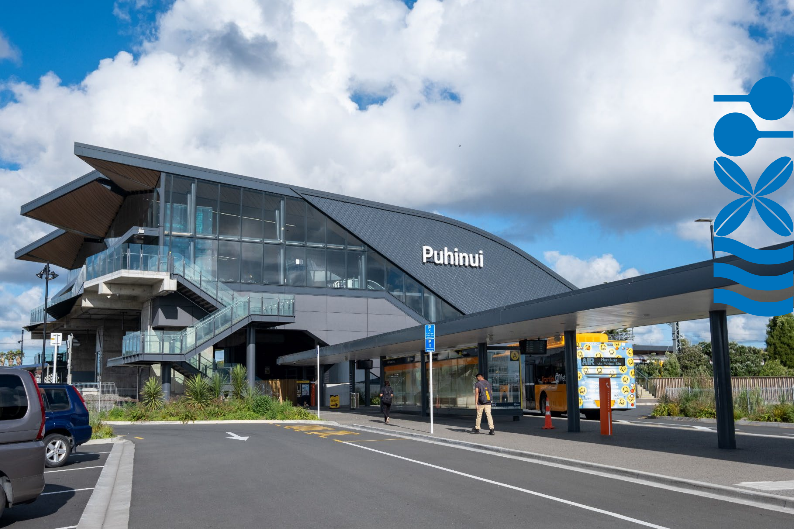
Puhinui Train Station
