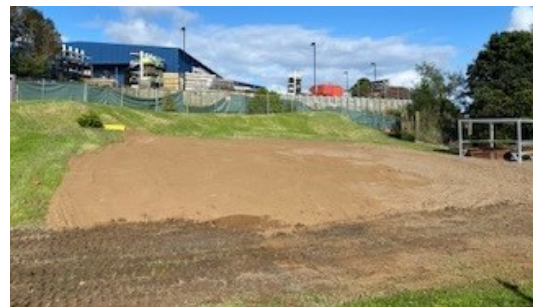
After – new exercise yard with levelled surface
