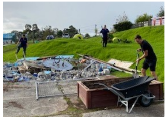
Before – old pool demolished and work starting
