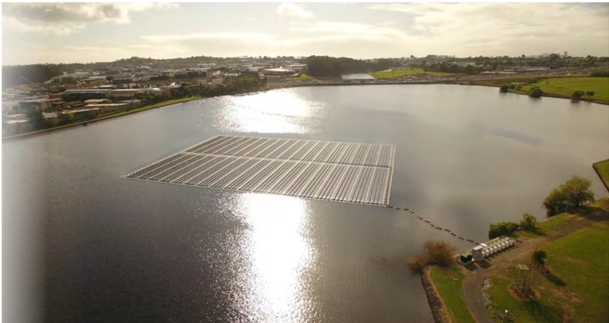
Floating solar array, Rosedale Wastewater Treatment Plant
