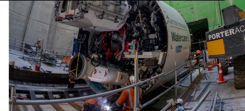
Domenica, a Micro TBM lifts the first pipe into the shaft at Watercare's Central Interceptor project site at May Rd, Mt Roskill.
