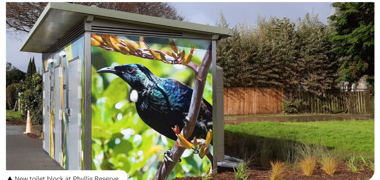
▲ New toilet block at Phyllis Reserve
