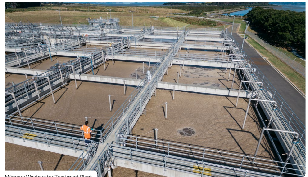
Māngere Wastewater Treatment Plant.
