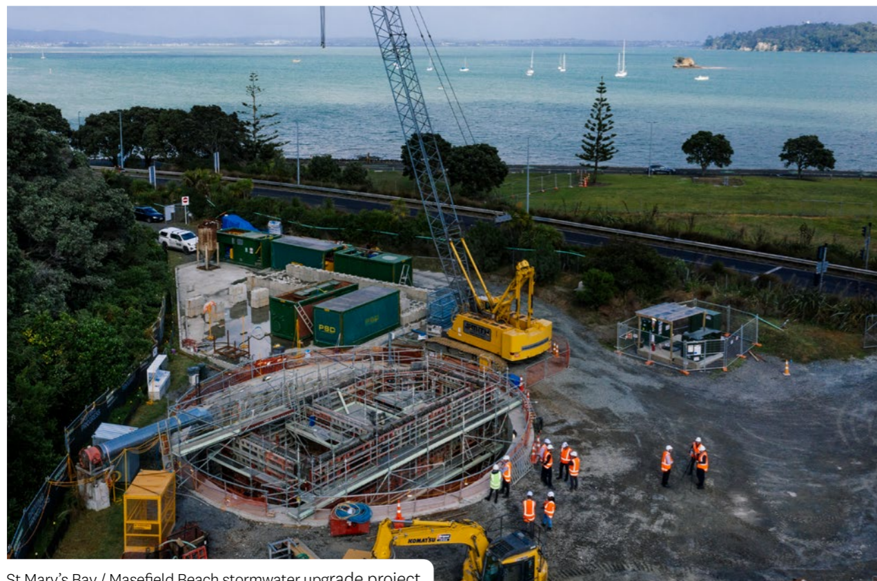
St Mary's Bay / Masefield Beach stormwater upgrade project
