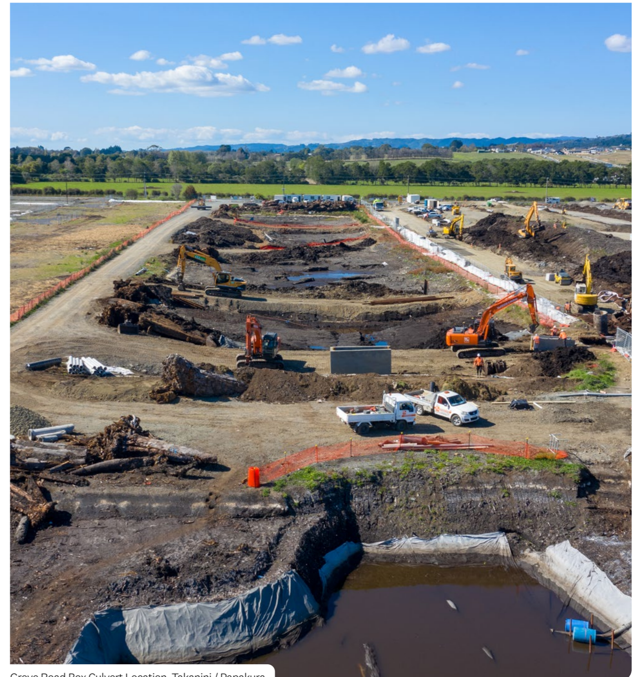
Grove Road Box Culvert Location, Takanini / Papakura
