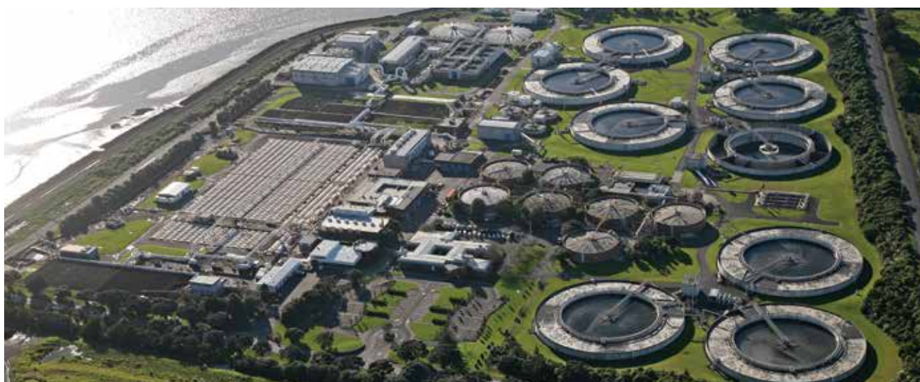
Aerial view of the Mangere Wastewater Treatment Plant where additional reactors will be constructed, to cater for Auckland's population growth.
