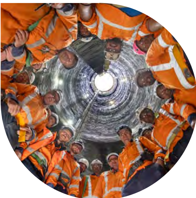
Central Interceptor crew at May Road branch sewer site
