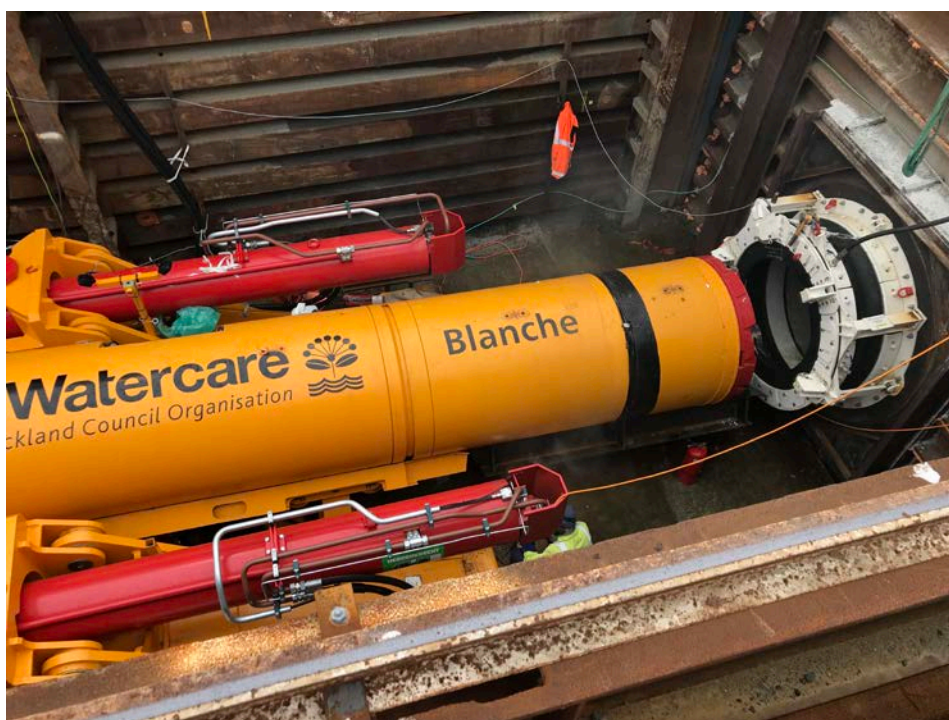
New tunnel boring machine, “Blanche”, Army Bay
