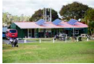
The local board funded installation of solar panels at Great Barrier Island Golf Club.
