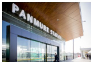
Panmure Train and Bus Interchange.
