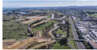
Development in the Bremner Road area, Drury.
