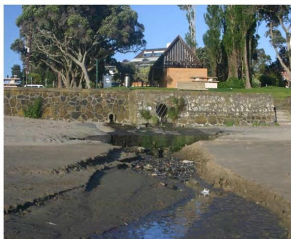
Figure 5.15 Coastal outfalls with erosion, Takapuna
