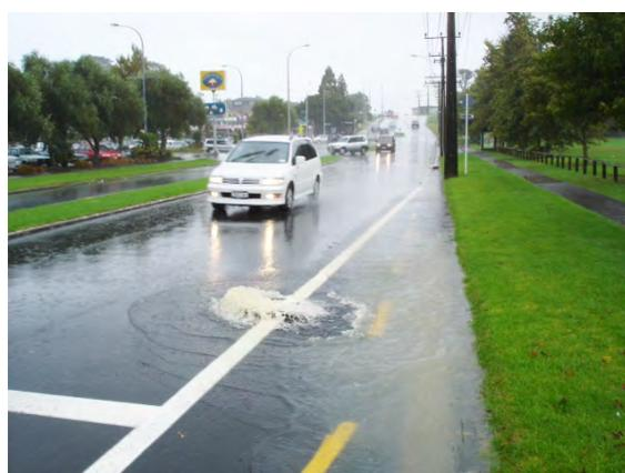
Figure 5.26 Surcharging Manhole, Northcote
