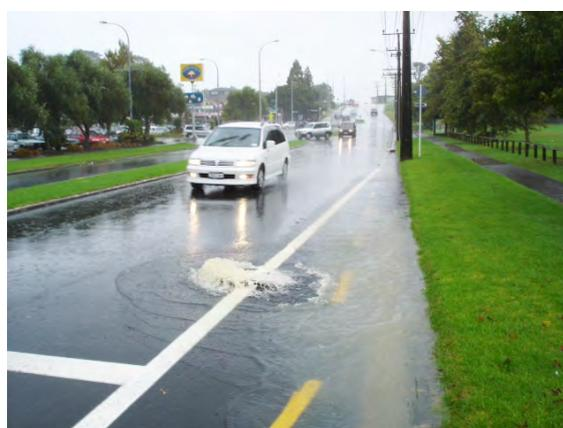
Figure 5.26 Surcharging Manhole, Northcote
