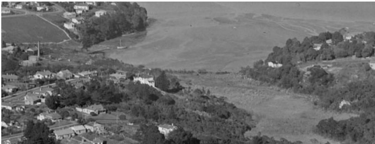
Figure 5: Historic aerial from June 1947 (Source: Whites Aviation)
