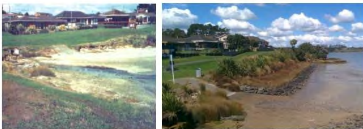
Figure 5-3: An eco-engineered hybrid approach to coastal protection along St Anne's Crescent in the Pahurehure Inlet. This case study featured salt marsh restoration, with the objective of providing weather protection to the sloping bank. Planted rushes landward of the bund aided in the protection to the bank and the provision of additional visual aesthetic values and functionality. Left. St Annes Crescent in 1993 (T+T, 2009). Right. St. Anne's Crescent salt marsh restoration. Note the planted vegetation between the foreshore and the rocky outcrops.
