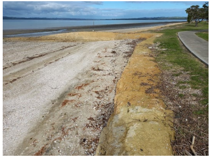
Figure 2-2: Shelly Beach Looking southward towards one of the mudcrete groynes. Native shells are visible in the seawall in the foreground.
