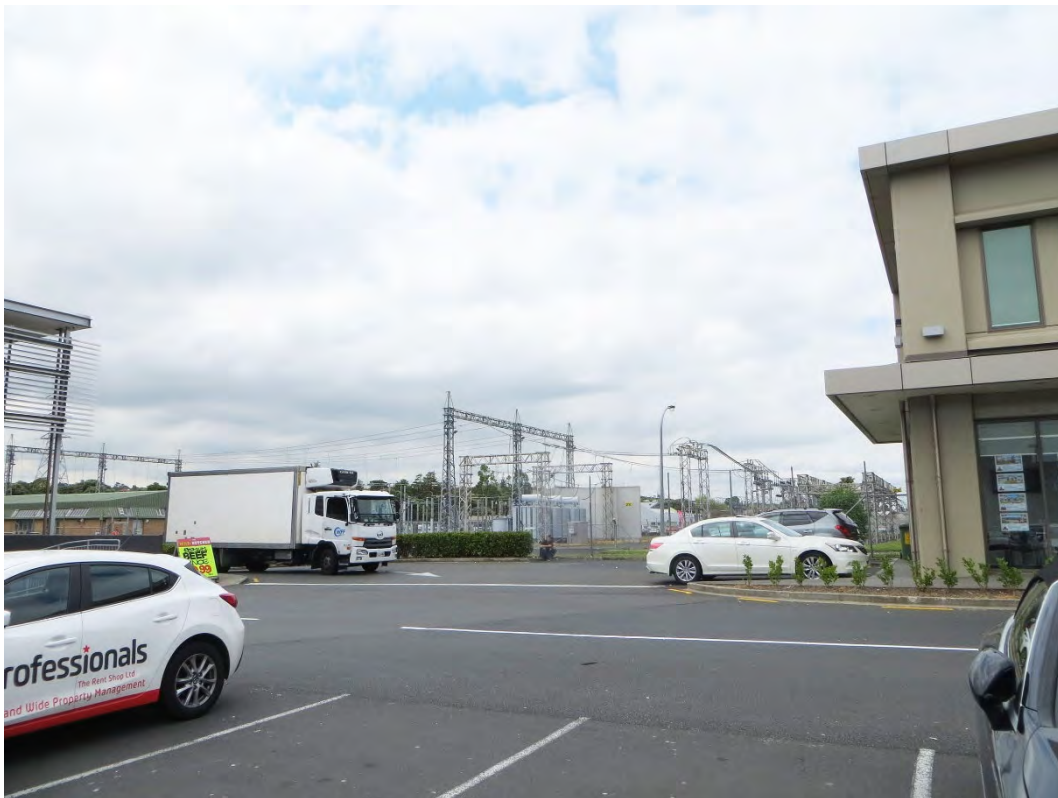
Photo 3: View from the retail complex car park to the north of the Wiri Substation Site, from where the Site's infrastructure is partially visible between the buildings.
