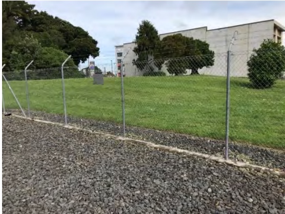
Figure 7 The location of the proposed switchroom buildings L and M and switchyard extension (looking north west)
