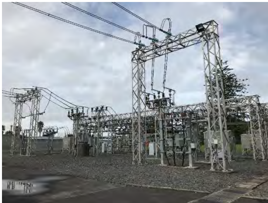
Figure 9 The existing 33kV switchyard to be removed (looking south west)
