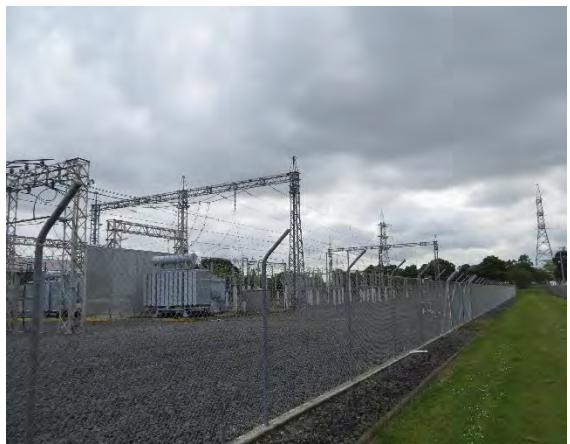
Figure 6 Existing 110kV gantries (view from south of The Site, looking east across the Site).
