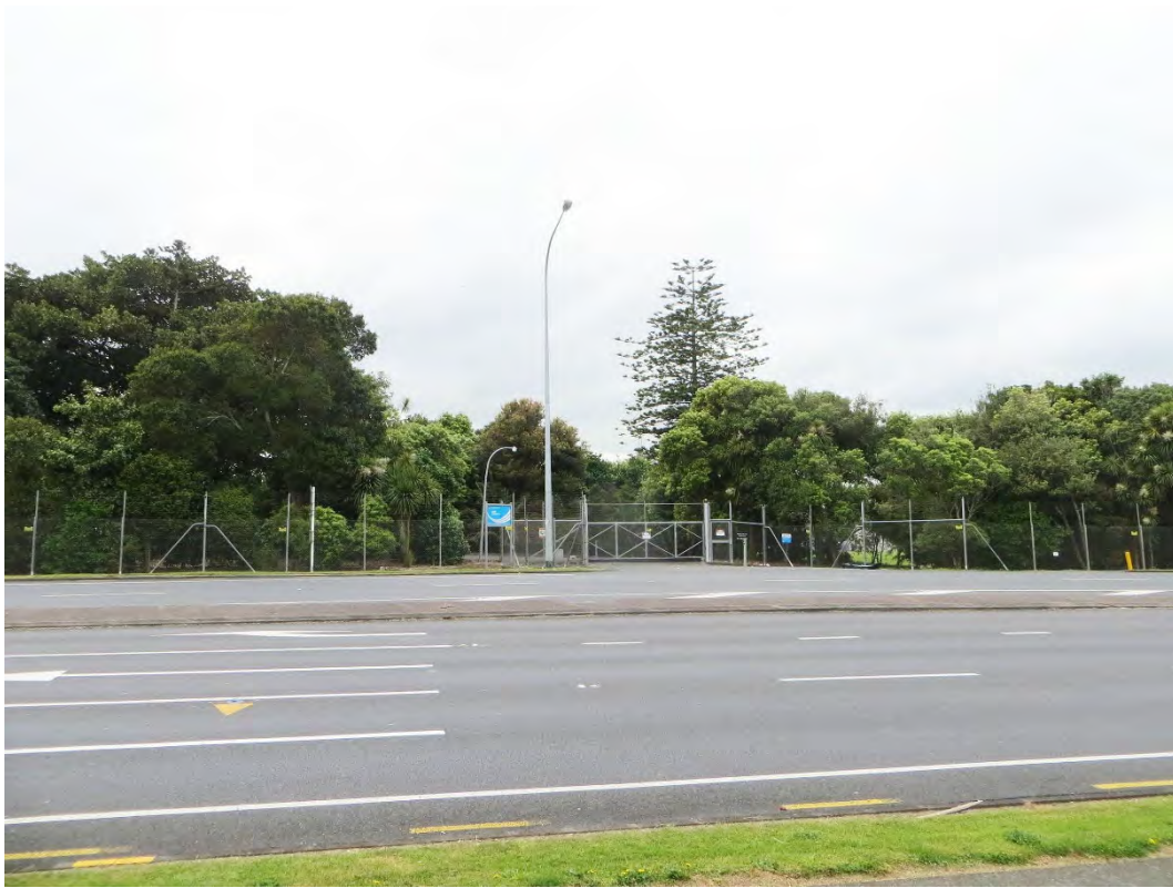
Photo 1: View from Great South Road opposite to the entrance gate of the Wiri Substation Site. View of the Site's infrastructure is screened by the intervening mature vegetation lining the Site's western boundary.
