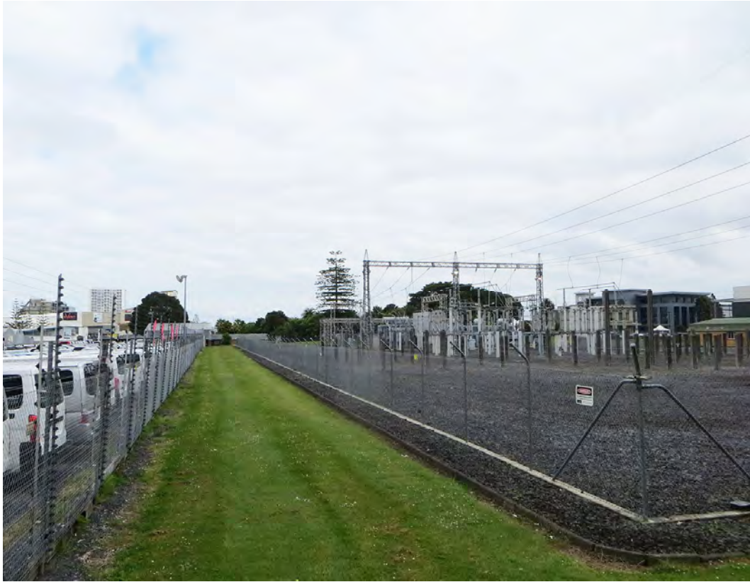
Photo 4: View from the Site's south eastern corner between the southern boundary abutting the car sales yard and security fence of the substation platform.
