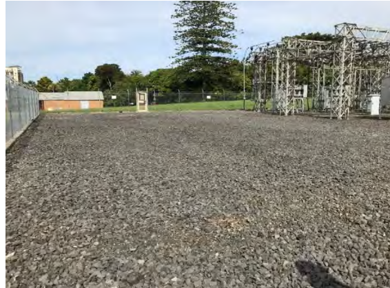
Figure 8 The location of the proposed switchroom building K (looking west)
