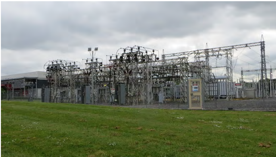
Figure 4 Existing 110kV switchyard and gantries at Wiri Substation (view from south looking north across the Site)
