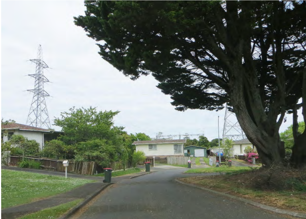
Photo 5: View from Seton Place, a street of residential housing to the east of the SH1 opposite to the Wiri Substation location.
