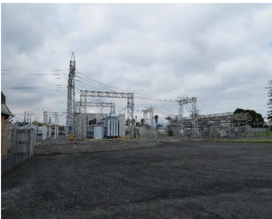
Figure 5 Existing 110kV and 33kV switchyard and gantries (view from north looking south across the site)
