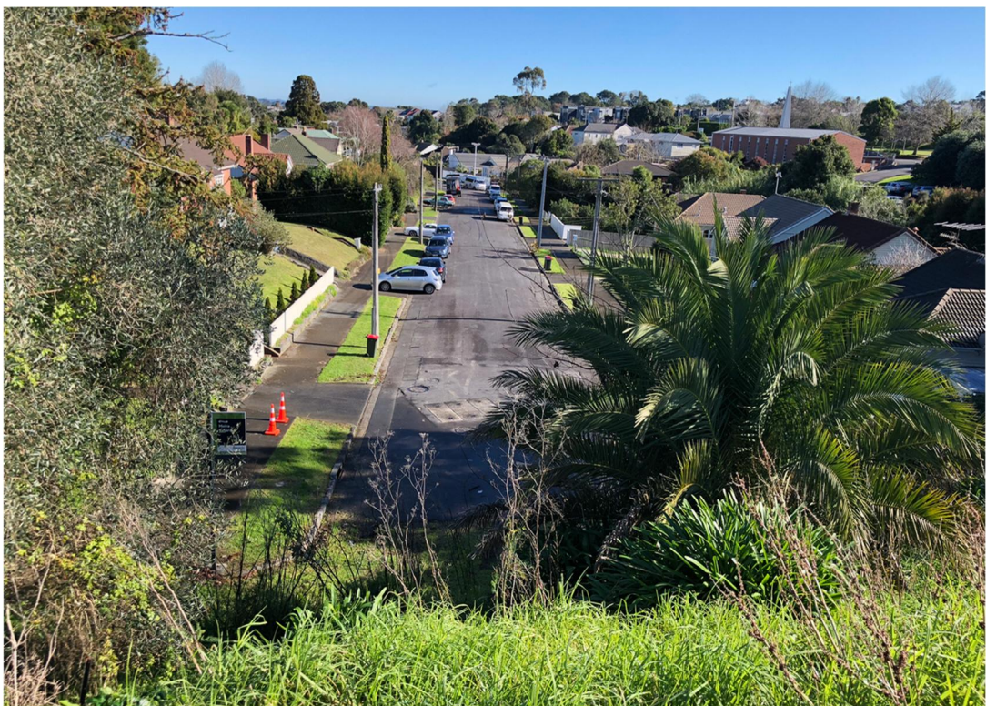
Figure 34. Looking west along Tawariki Street from the raised sports fields of St Paul's College
