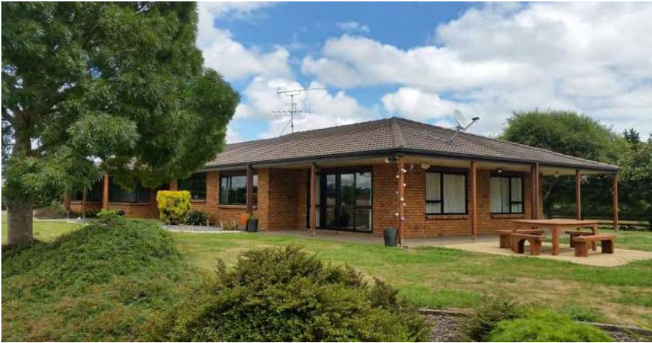
Western Curtilage Area - Dwelling (2)
