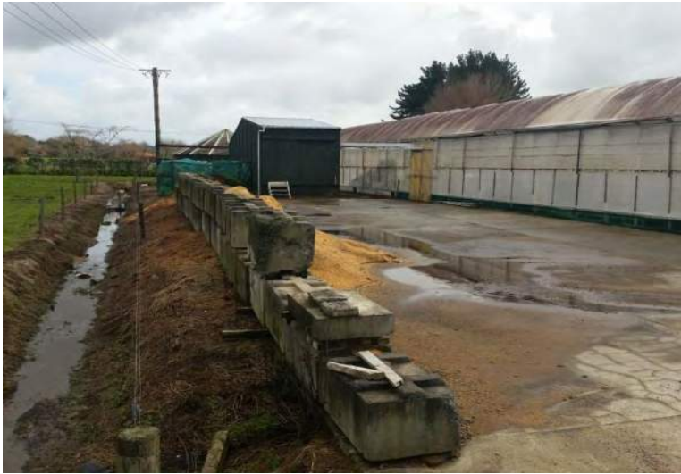
Mixing shed and water tank
