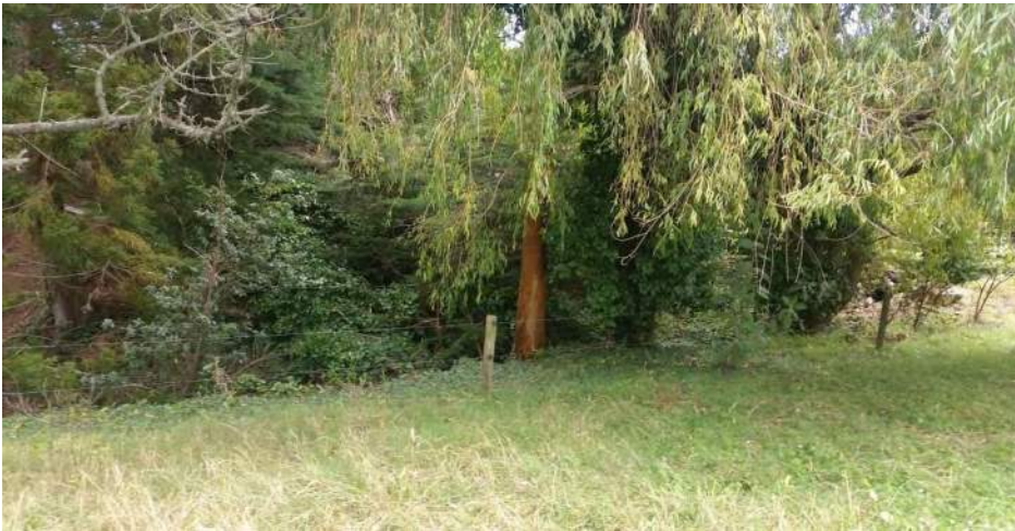
Central Gully and Culvert
