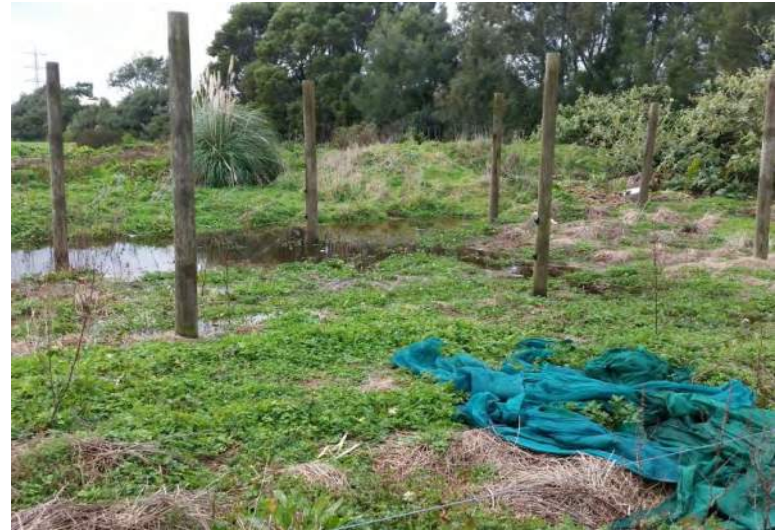
Stockpiled fill materials
