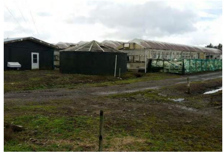
Packhouse, water tank and greenhouse
