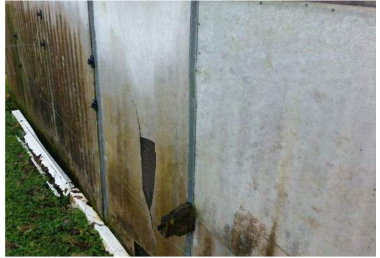
Suspected asbestos containing materials
