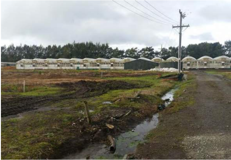
Greenhouse, mixing and pump shed and water tank
