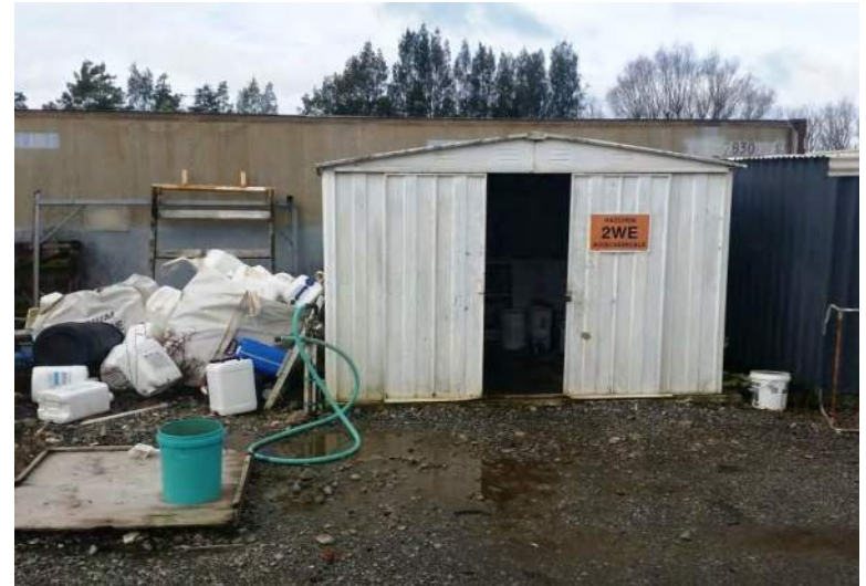
Chemical storage shed
