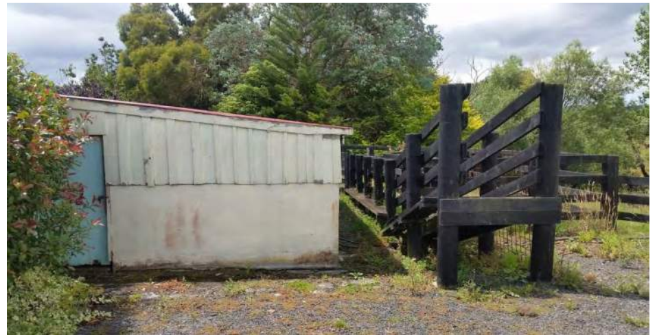
Stock Loading Yards and Auxiliary Shed (2)
