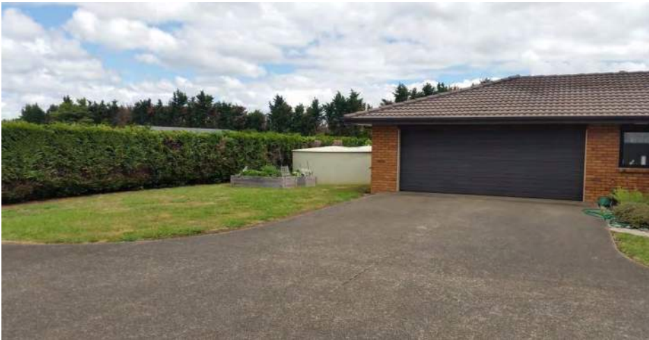
Southern Curtilage Area - Dwelling (2)
