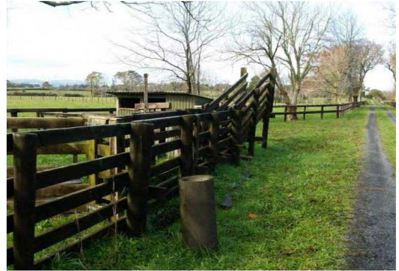
Stock loading yard
