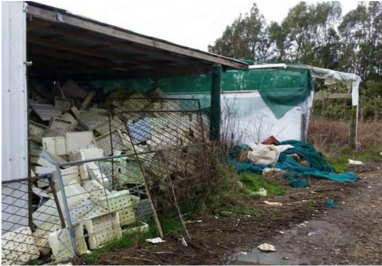
Additional storage sheds
