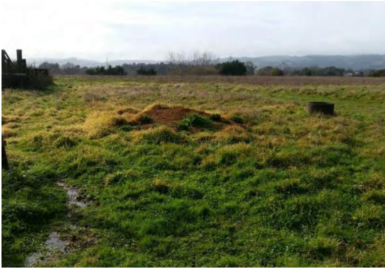
Stockpiled fill material (SP01)
