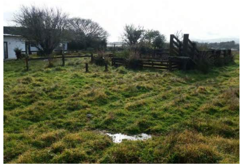
Stock loading yard
