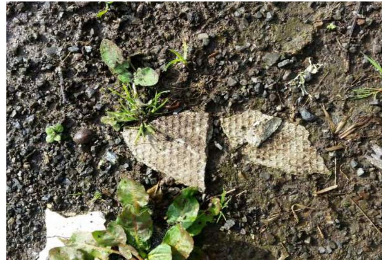
Evidence of asbestos
