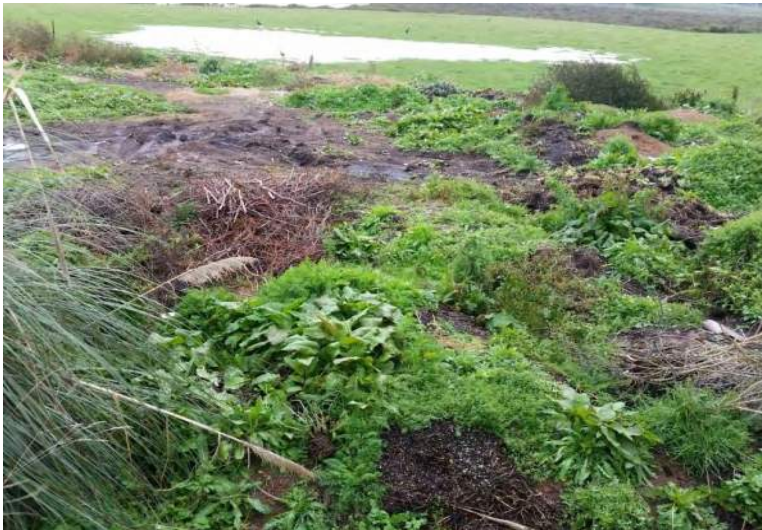
Stockpiled fill materials
