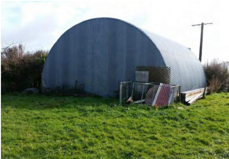
Storage surrounding barn
