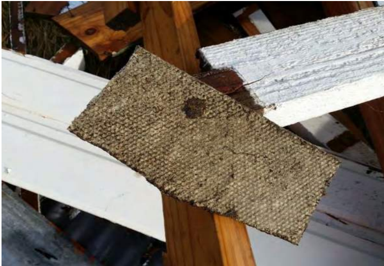
Evidence of asbestos
