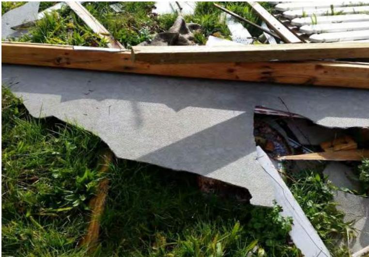
Evidence of asbestos
