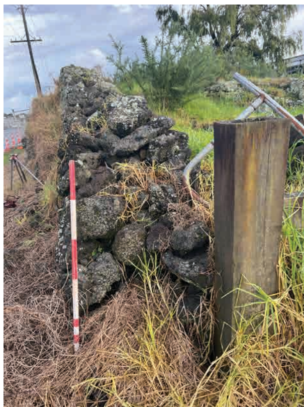
Figure 5. West facing view of drystone walls, showing internal structure.
