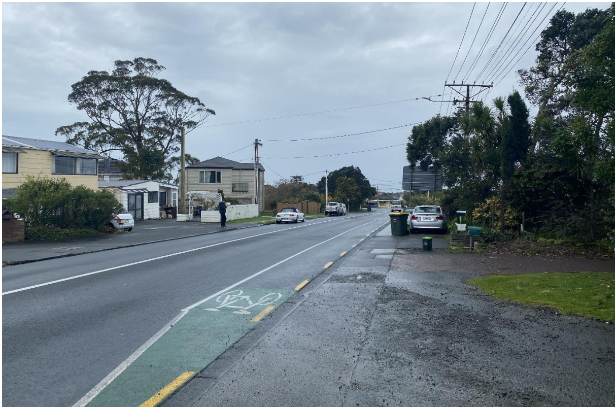
Photograph 5: Available sight distance to the east of the existing access along Browns Bay Road
