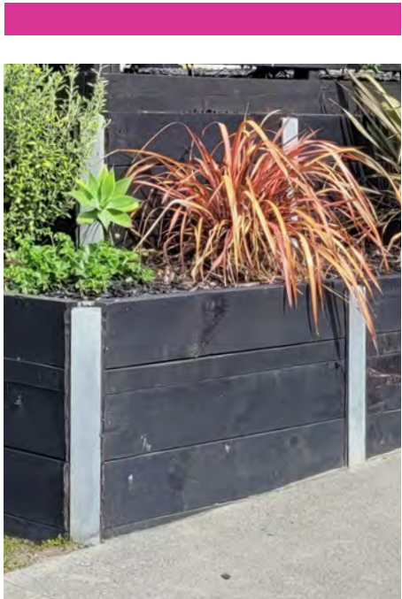
TIMBER / STEEL BEAM RETAINING WALL
