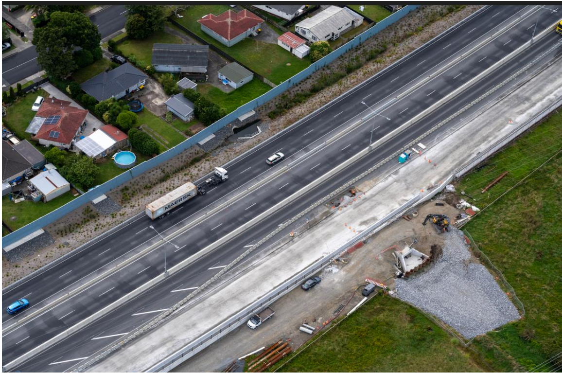
Figure 3: Aerial photos showing construction of the culverts
