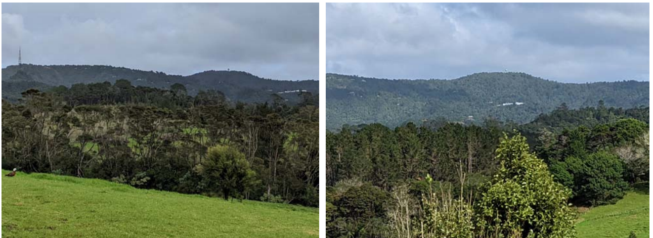
The Radome visible from #8 Gum Road, left and #101 Coulter Road, right
