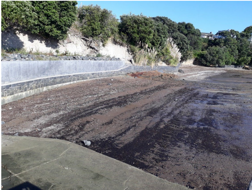
Figure 37: Mass concrete retaining wall (Auckland Council asset) constructed at Andersons Bay, Glendowie (Source: Auckland Council)
