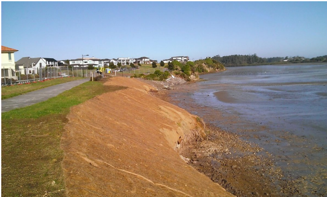
Figure 42: Karaka Harbourside esplanade reserve following removal of undermined tree stumps and re-grading of cliff edge in 2015 (Source: Auckland Council)
