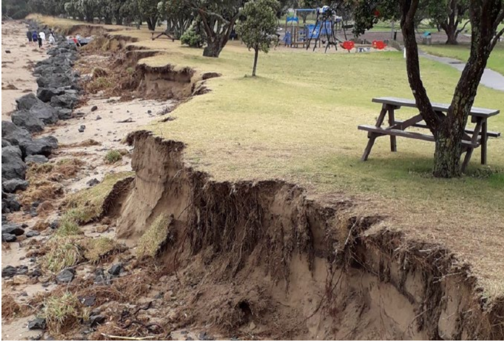
Figure 9: Coastal erosion at Stanmore Bay, Whangaparāoa following January 2018 storm events. The event lowered beach levels, exposing legacy buried rock and eroding the reserve edge (Source: Auckland Council)
