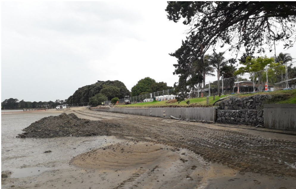
Figure 36: Repairing of an existing failing seawall along the western end of Sandspit Beach. (Source: Auckland Council)
