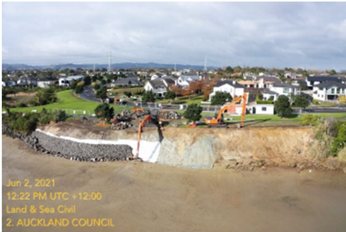
Figure 46: Karaka Harbourside - Stage two rock revetment, completed in 2021 (Source: Land & Sea Civil Ltd)
