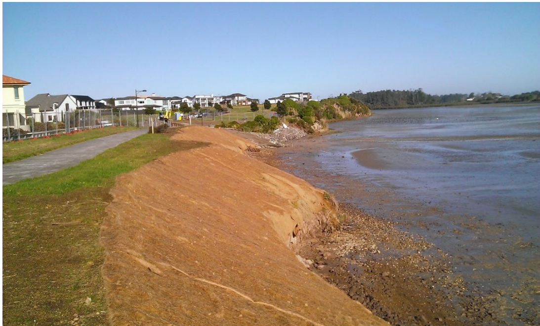
Figure 22: Karaka Harbourside esplanade reserve following removal of undermined tree stumps and re-grading of cliff edge in 2015 (Source: Auckland Council)
