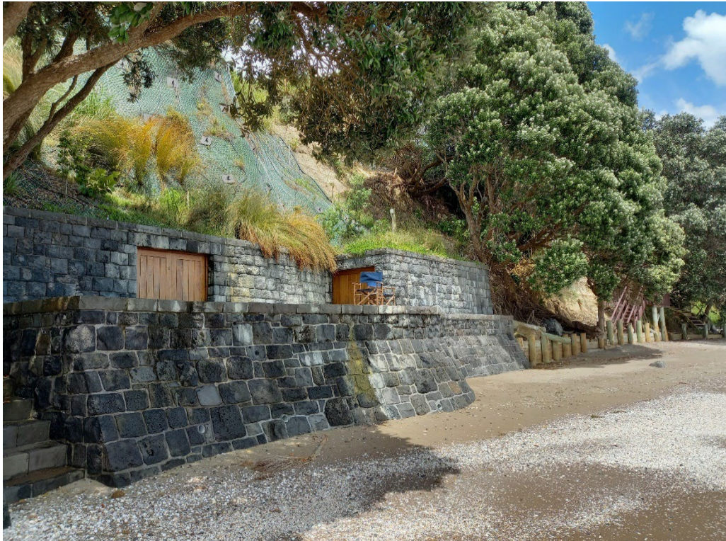
Figure 38: An example of soil nails and hard coastal protection structure at Beachlands (Source: Auckland Council)
