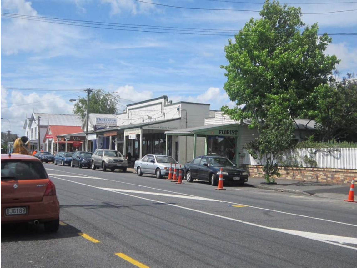
Figure 4: The buildings at 128-140 Hinemoa Street as seen from the north. At the far end of the row is 140 Hinemoa Street, scheduled in the district plan for its heritage values.
