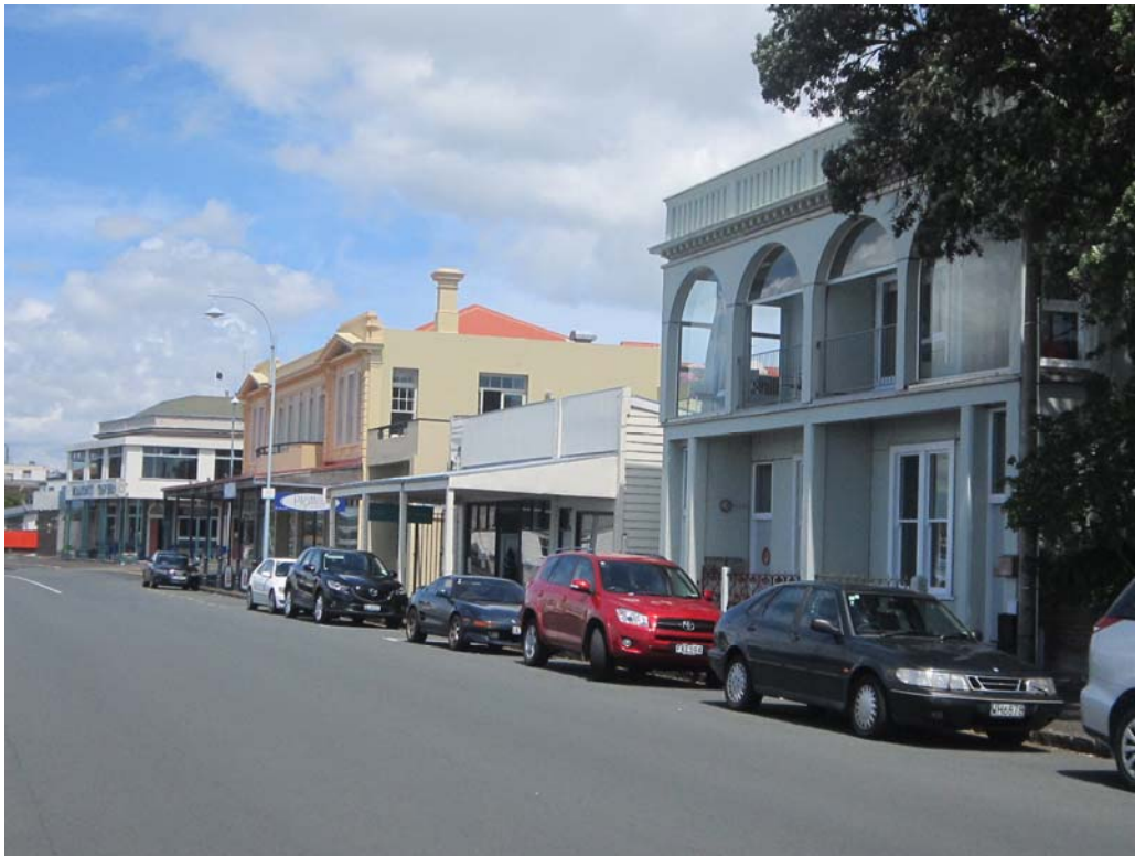
Figure 10: Buildings at the intersection of King Edward Parade and Church Street. At the far left is the Masonic Tavern at 29 King Edward Parade. The single-story commercial building at 35 Kind Edward Parade retains original shop-front joinery.
