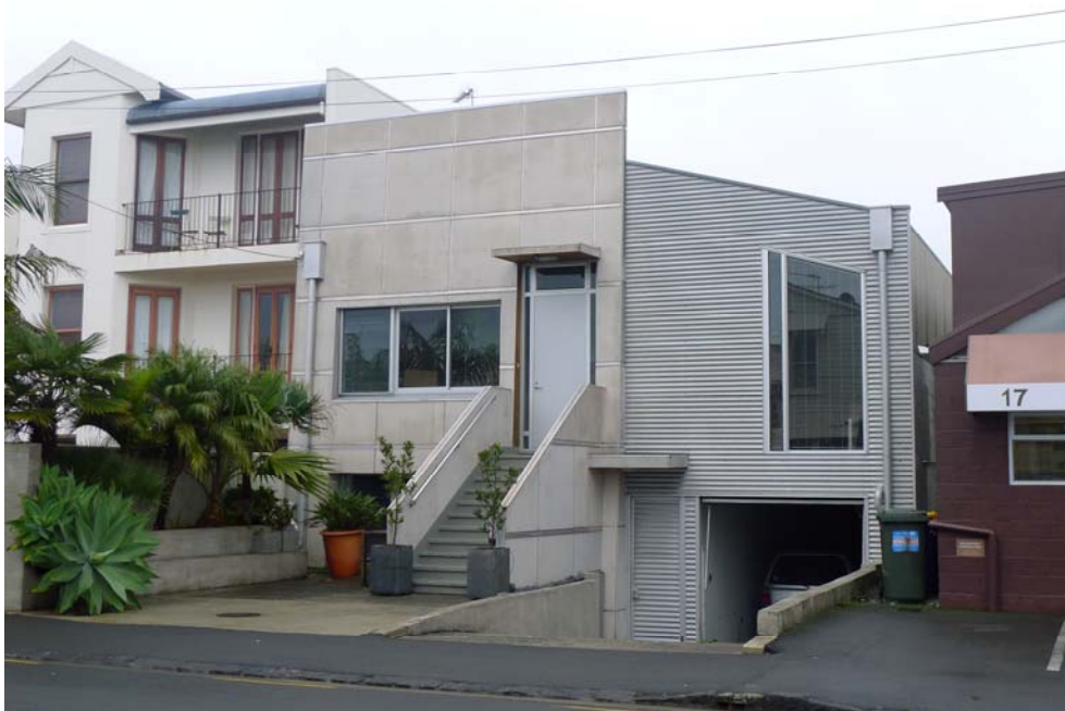
Figure 6: A new addition to Wynyard Street which is entirely of today in terms of its design, but which successfully responds to the industrial aesthetic of its context. To the left is a 'pastiche' style development which is considered to be less successful in that it is a contrivance which does not belong either in a historic period or today.
